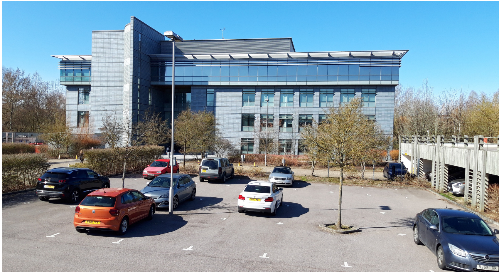
Existing Site Photo
