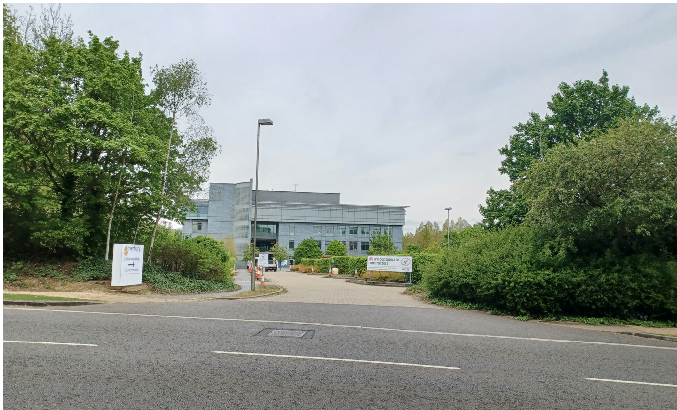
View from roadside (Brook Drive)
