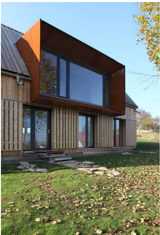
◇ CHAMFERED CORTEN DORMER WINDOW
