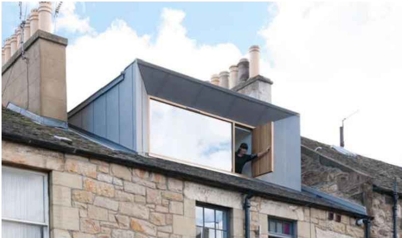
◇ CHAMFERED ZINC CLADDED DORMER WITH TIMBER INSERTS
