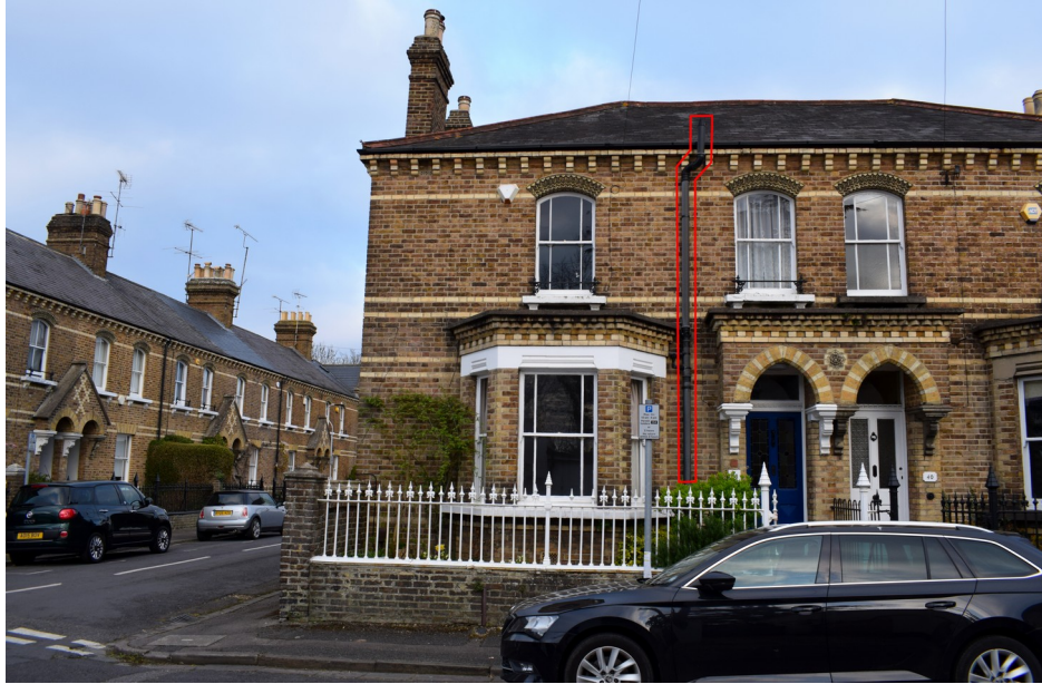
Front elevation showing existing downpipe - to be removed
