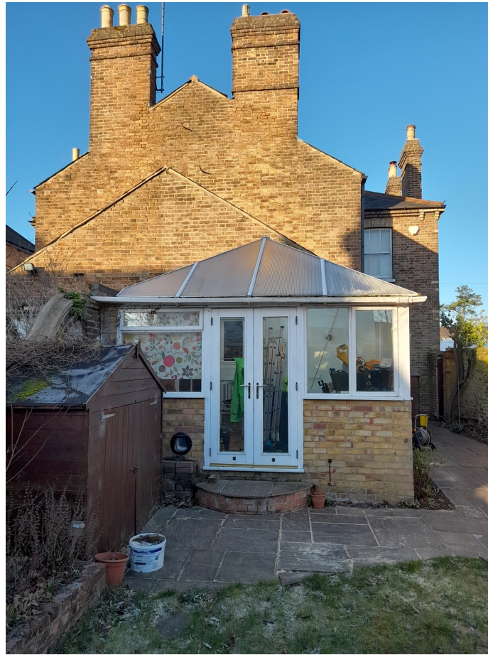
Rear view as existing
