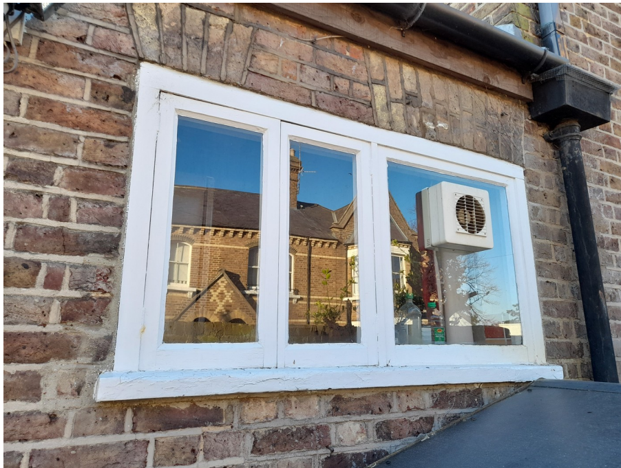
Non-original kitchen window
