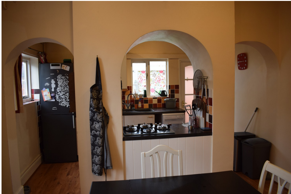
Modern arch topped openings between existing kitchen and dining areas
