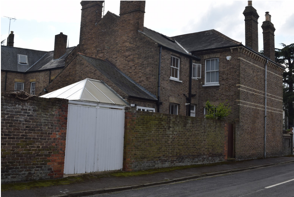
Rear view from the street
