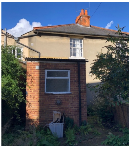
Plate 3: Rear elevation of No.35 with brick built single-storey extension
