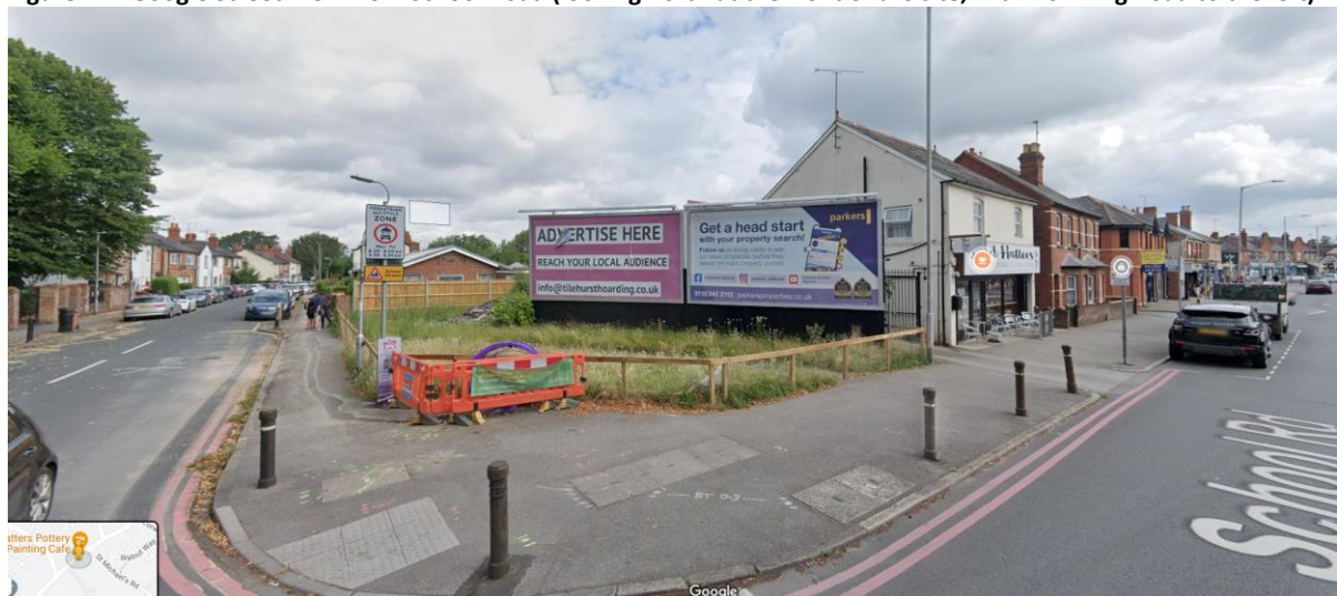
Figure 2.2: Google Street View from School Road (looking north at the front of the site, with Downing Road to the left)
