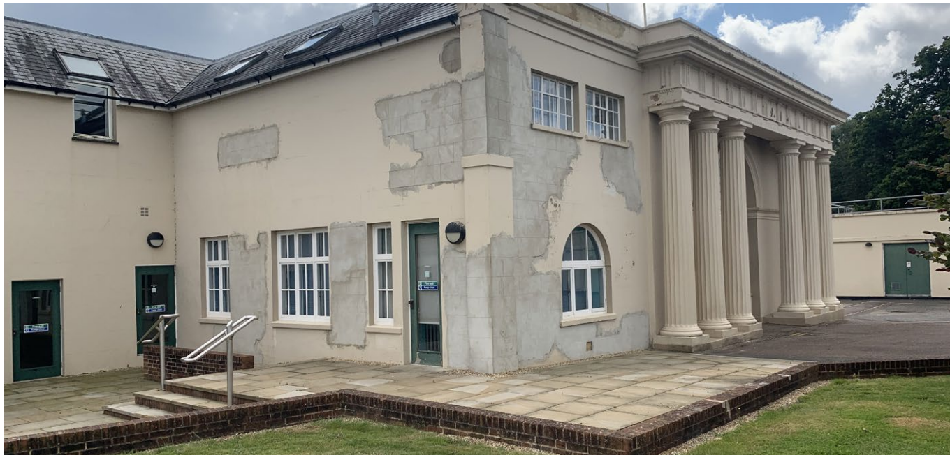
Recent repairs to the external fabric
