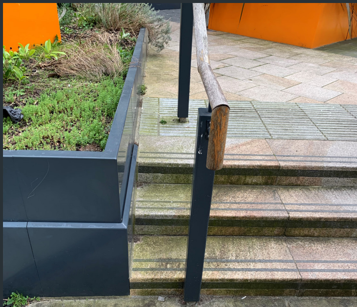
Existing planters alongside the handrail and level change
