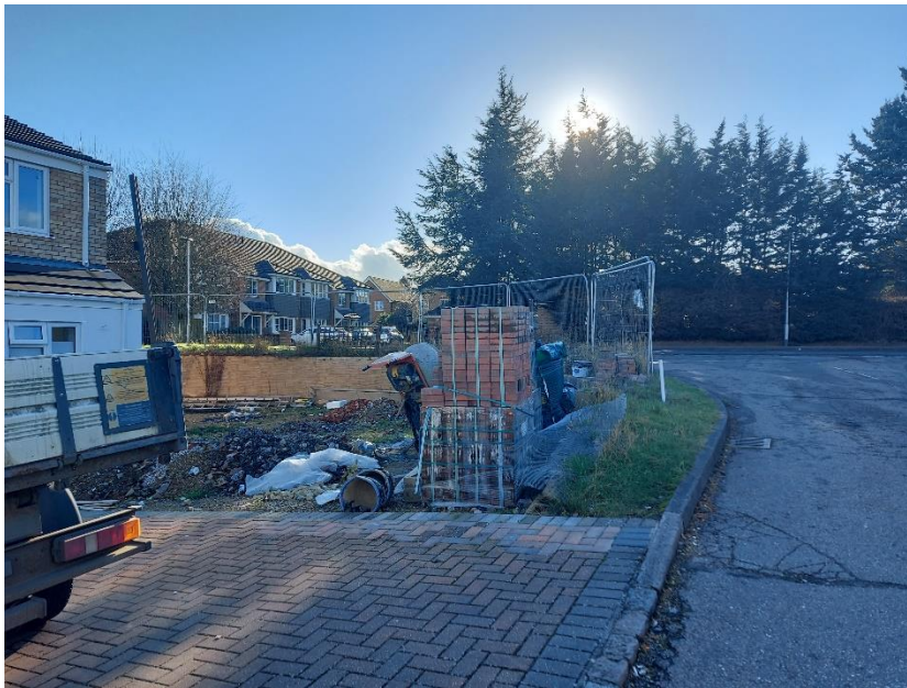
1 Application site photo taken at site visit on 24/02/2022
