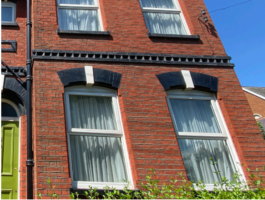
Figure 17 Existing brick and detail of window fenestration
