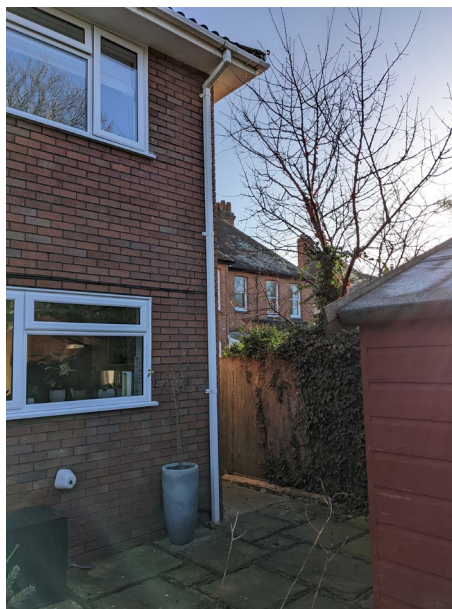
4.0 Neighbouring property south boundary
