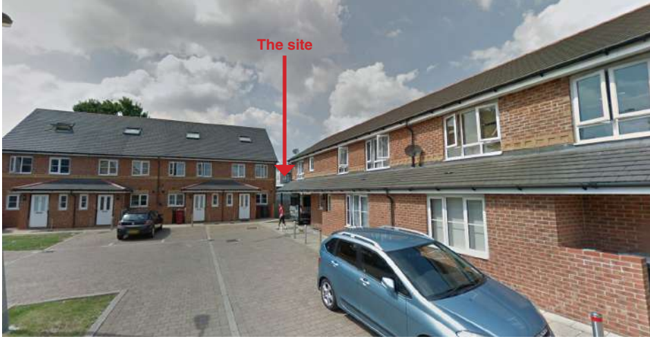
4. View of Battle Place which backs on to east boundary the proposed development site
