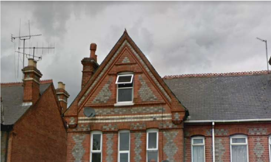
4. Oxford Road Houses - Recessed brick work
