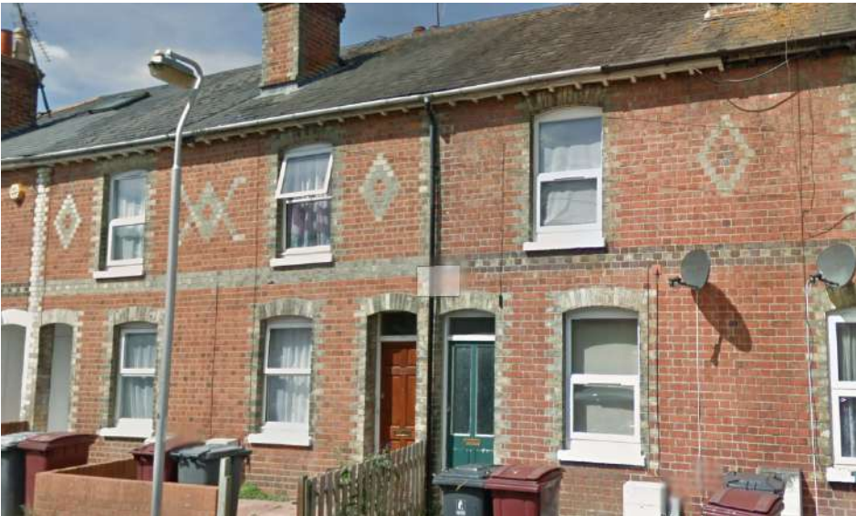
7. Feature brick work
