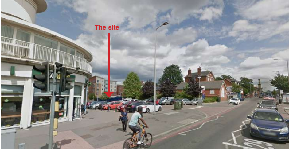
5. The site looking north east as viewed from Oxford Road.
