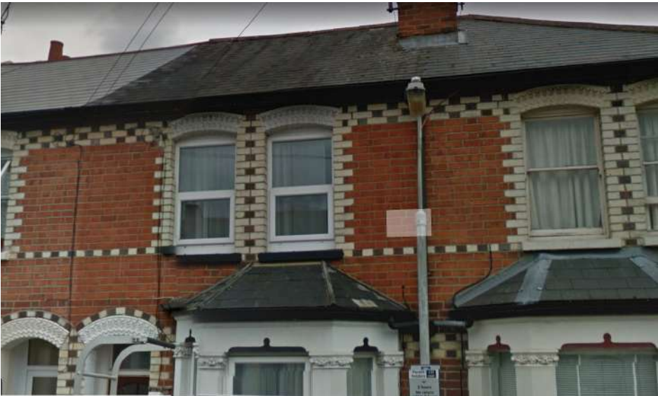
2. Nearby Terrace Housing - Feature brick banding
