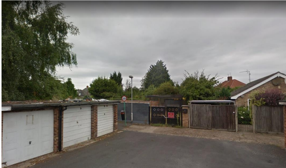
16 Byworth Close to the right, with the access gates to the application site on the left
