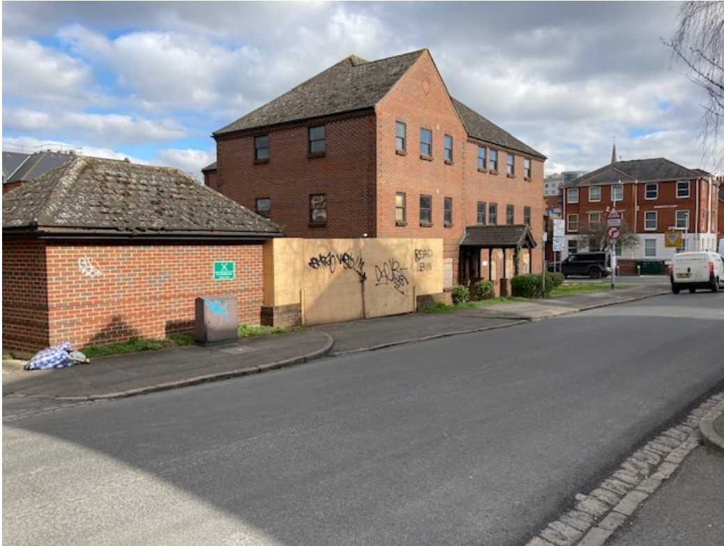
Photograph 2: the existing buildings and access onto South Street.
