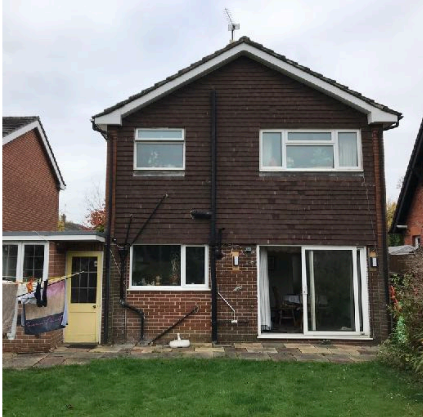
Rear view (east elevation) of the site; there is an inadequately constructed side extension with garage and wc / stores, which is uninsulated, and the kitchen is small and does not allow for modern family living
