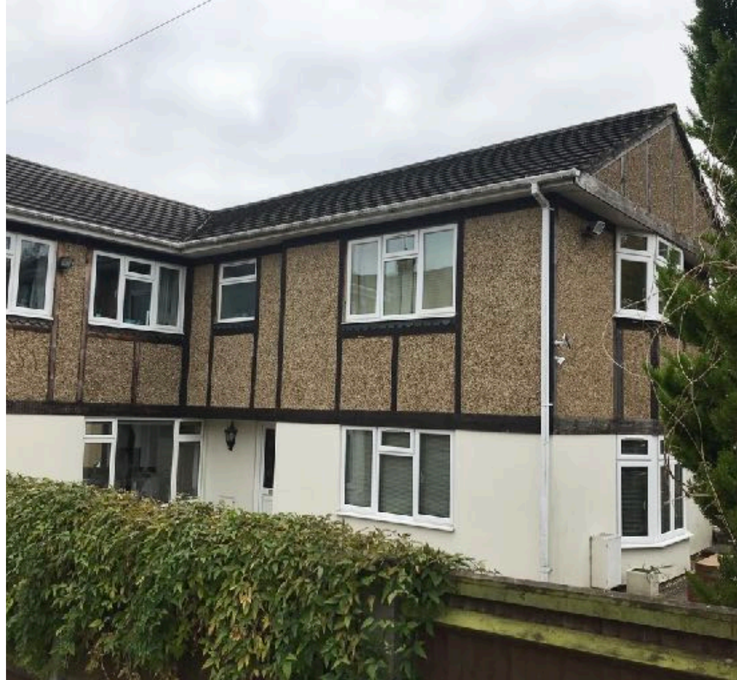
Front view of the property including the large 2 storey extension to the front of the original part of the house
