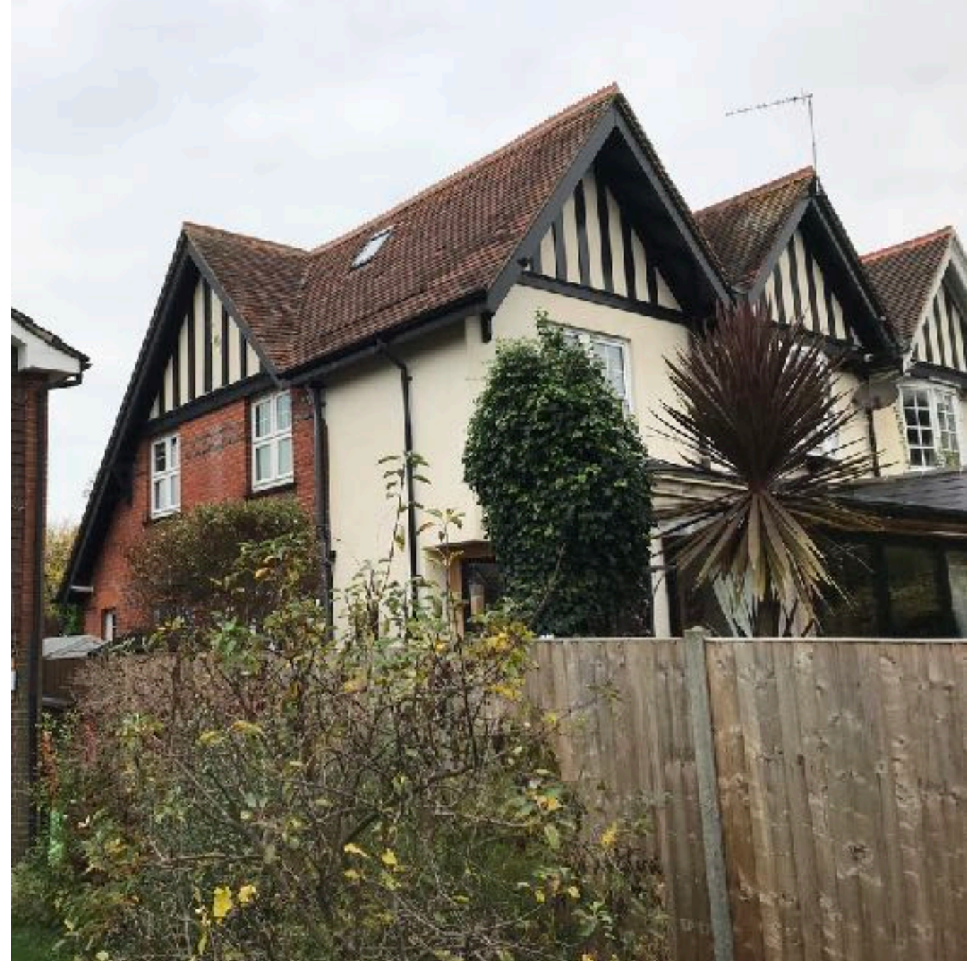
The rear extension with traditional gable to match the existing gable, and ground floor extension just visible at 85 Berkley Avenue
