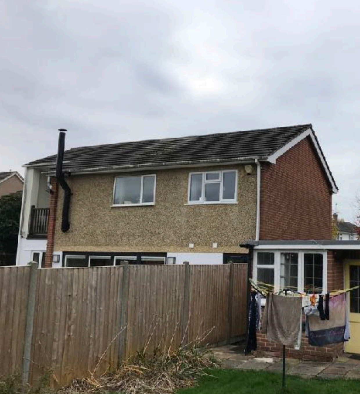
Rear view of 7 Ashley Road, which was constructed at the same time as the application property
