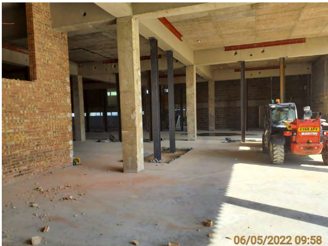
Plate 2 - Looking northwest from central Eastern loading bay.
