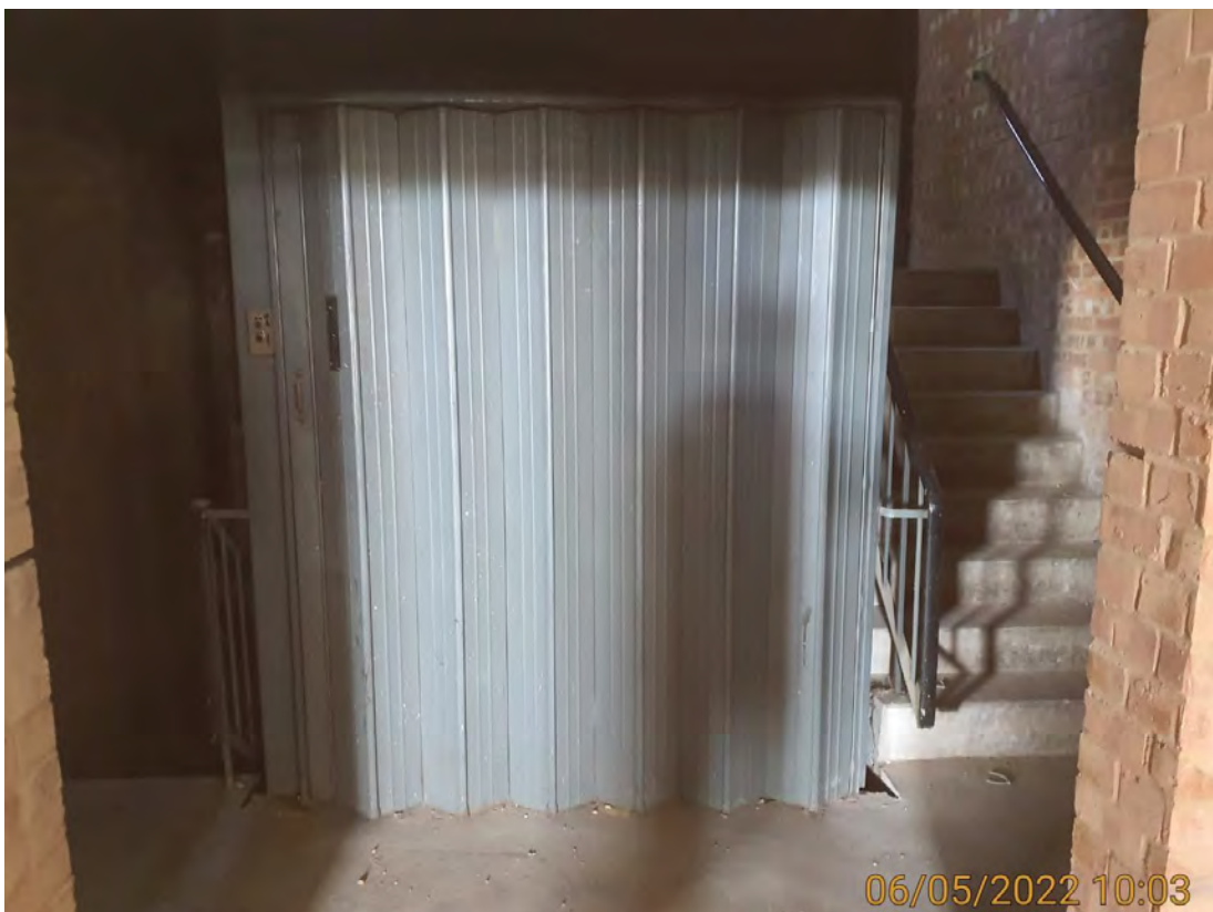
Plate 4 - Interior stairwell in the west of the building.
