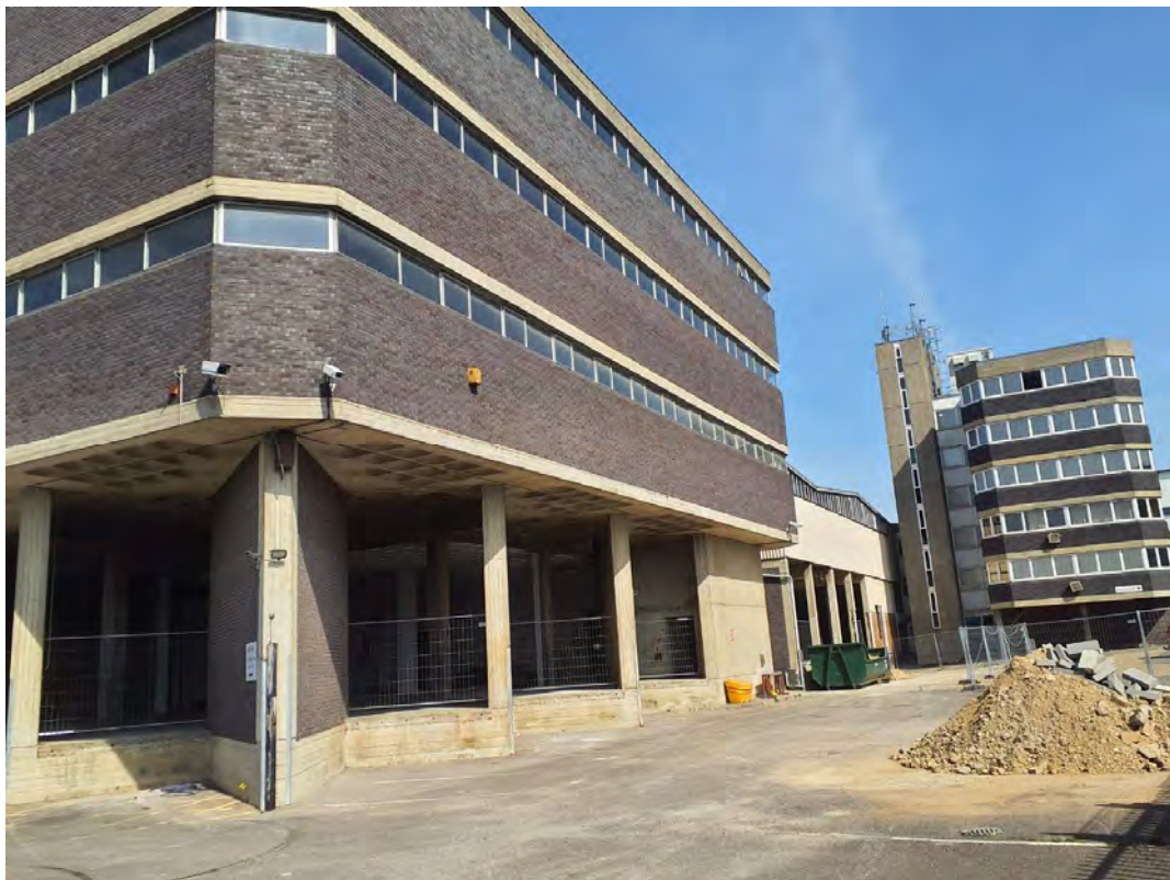
Plate 22 - Three story to five story building disused offices overlying large storage area with loading bays.
