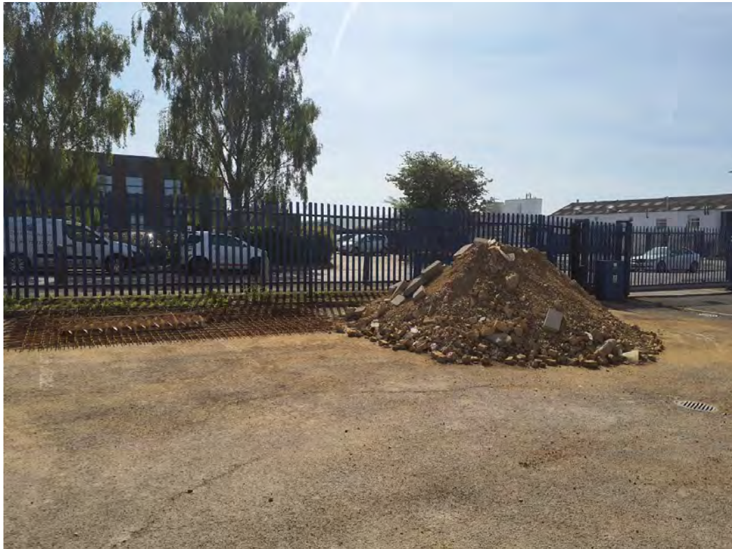
Plate 17 - Brick and concrete rubble alongside rebar mesh located in the east of the site.
