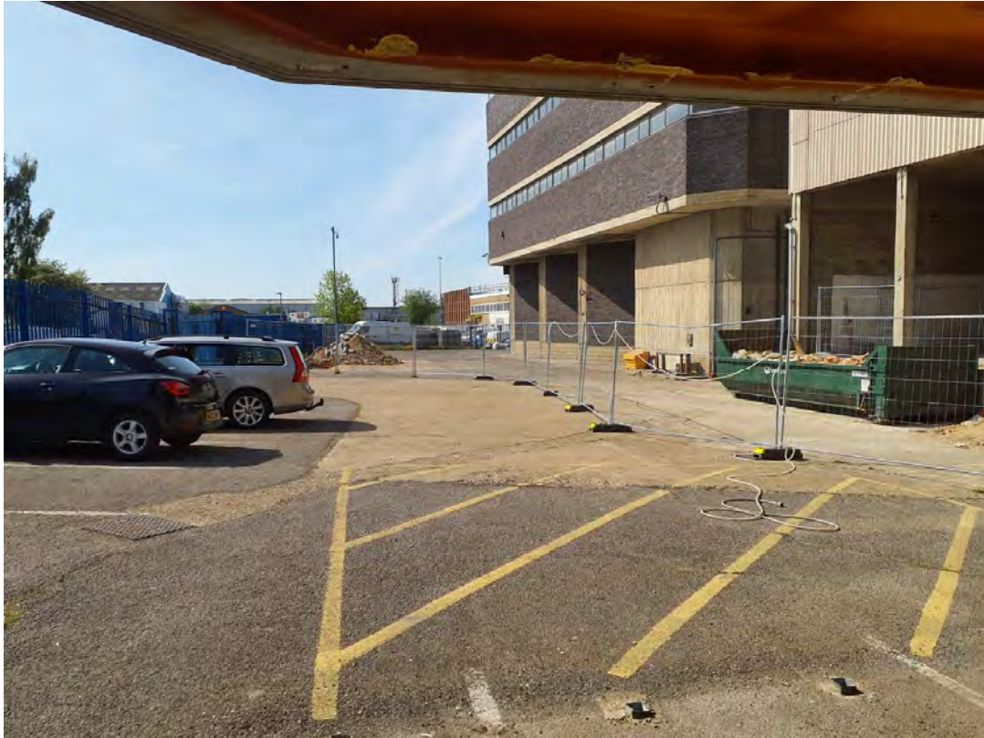
Plate 33 – View from the north of the site facing south.
