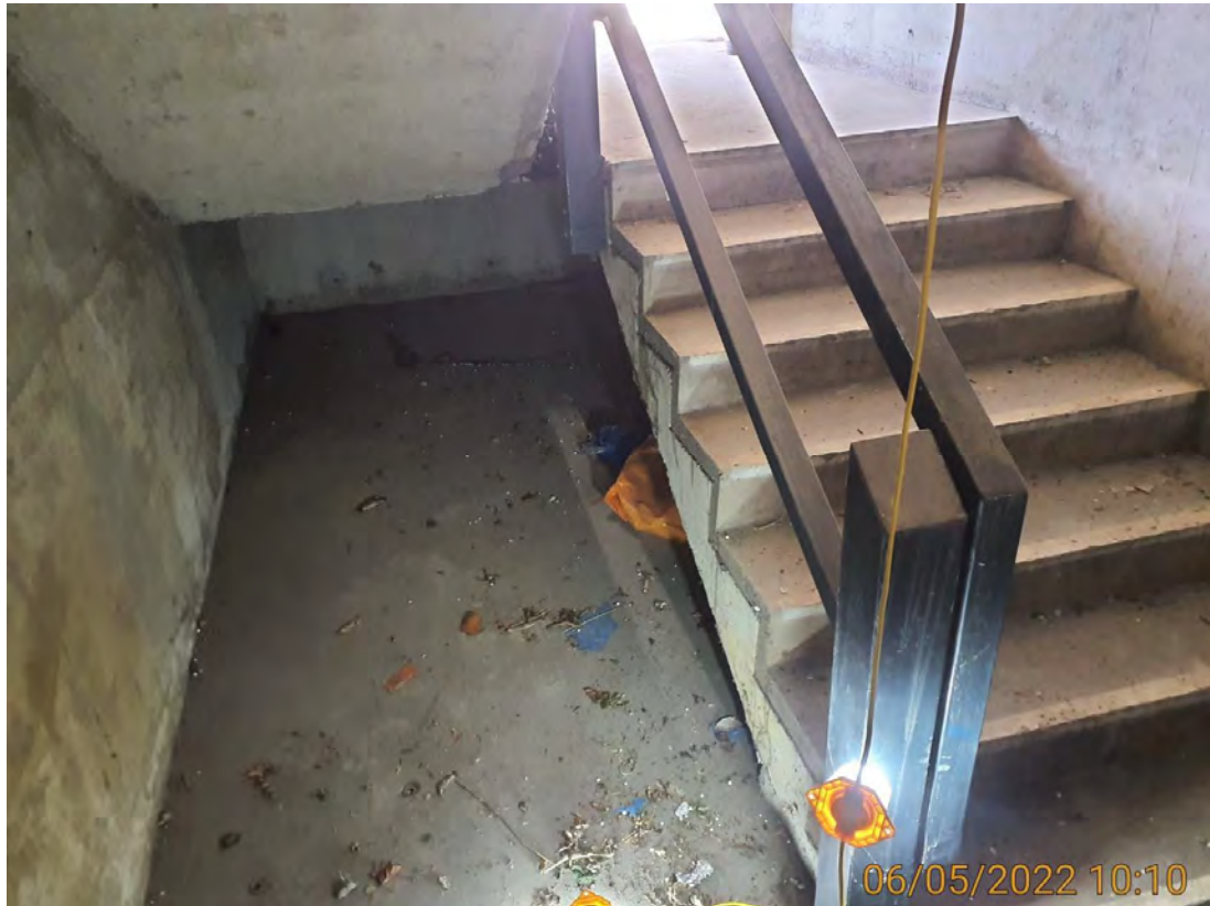
Plate 13 - Lowest level within the central Eastern stairwell.
