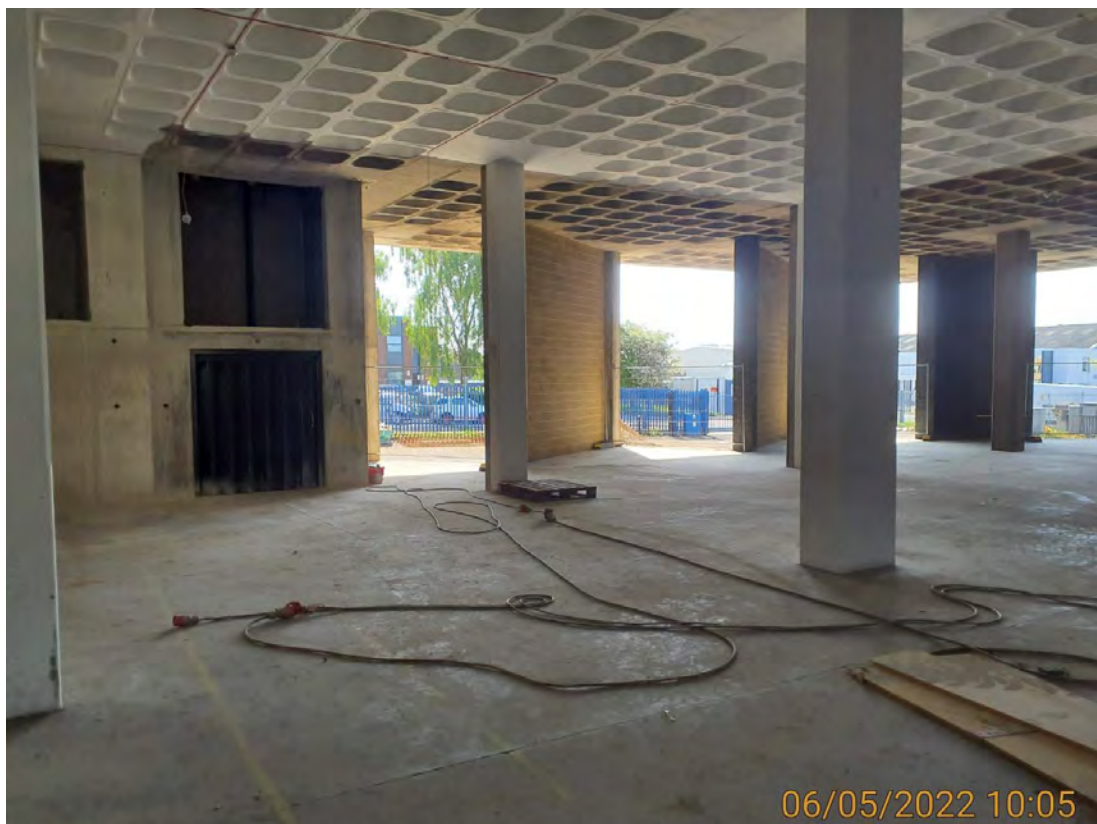
Plate 6 - Looking out to the southeast loading bays.
