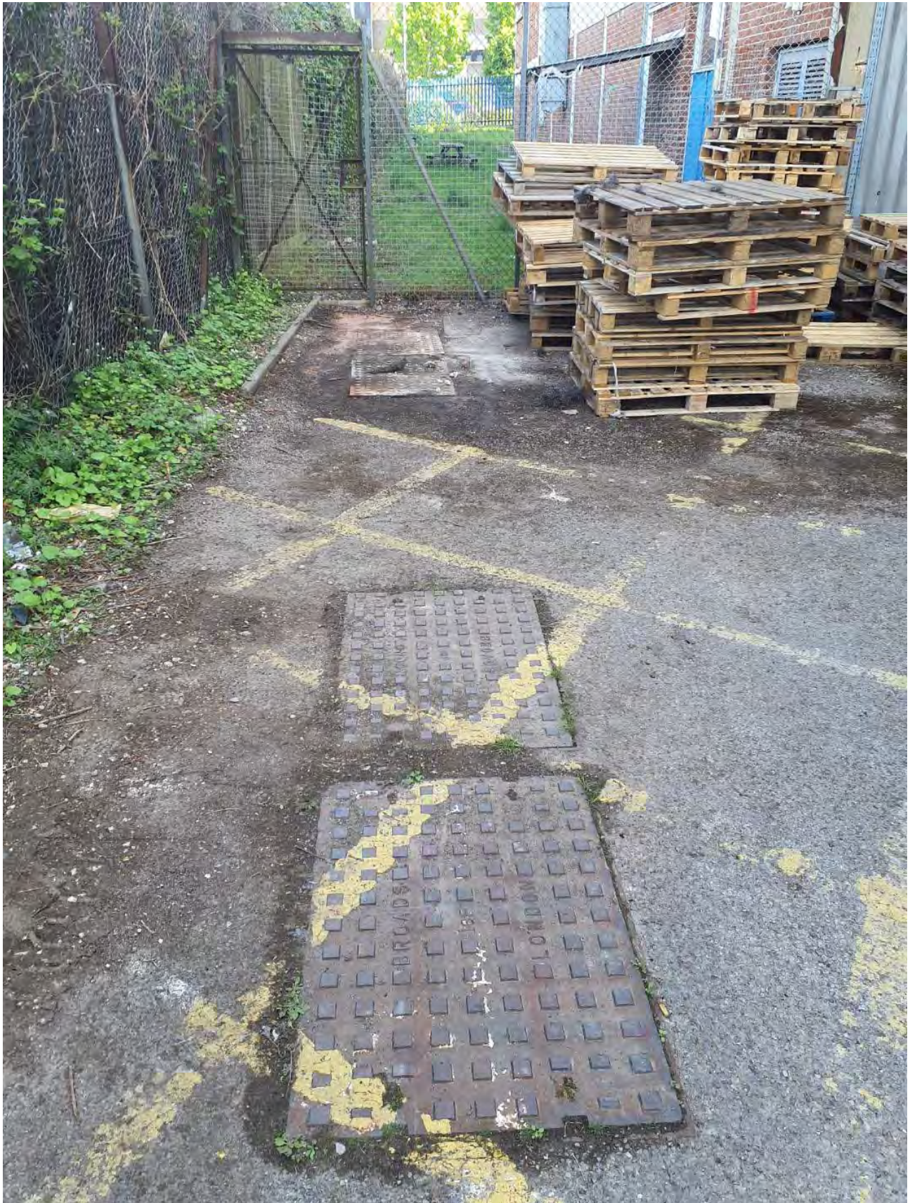
Plate 25 - Additional manhole covers in the Western portion of the site
