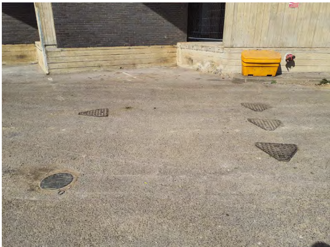
Plate 16 - Manhole covers and drains located in the central Eastern portion of the site.
