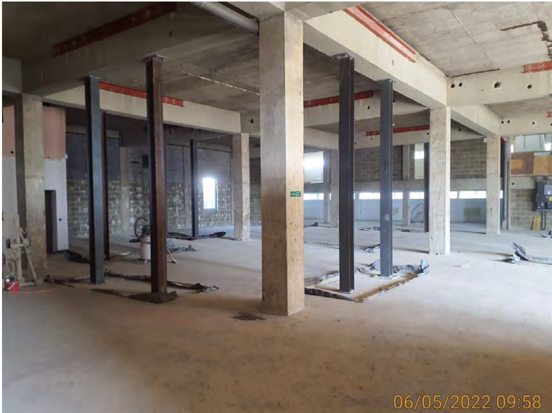
Plate 3 - View into the back of the loading bay (behind brick wall).
