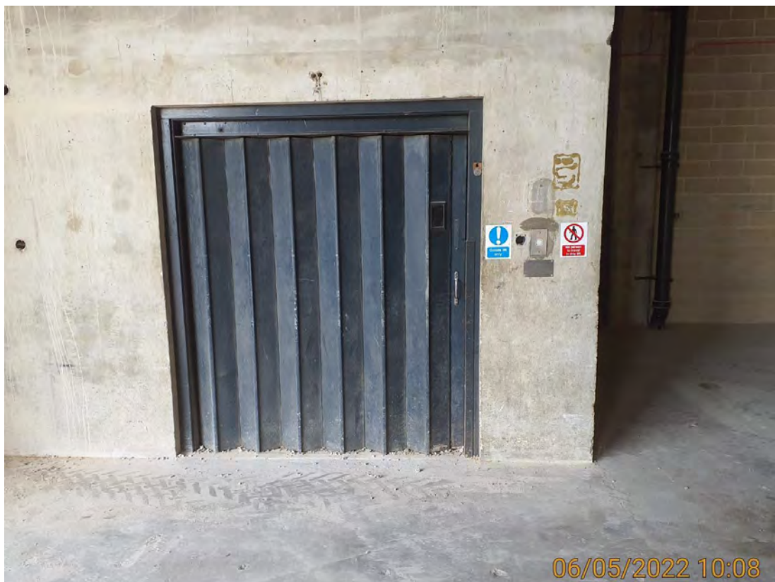
Plate 10 – Goods lift adjacent to southwestern stairwell.
