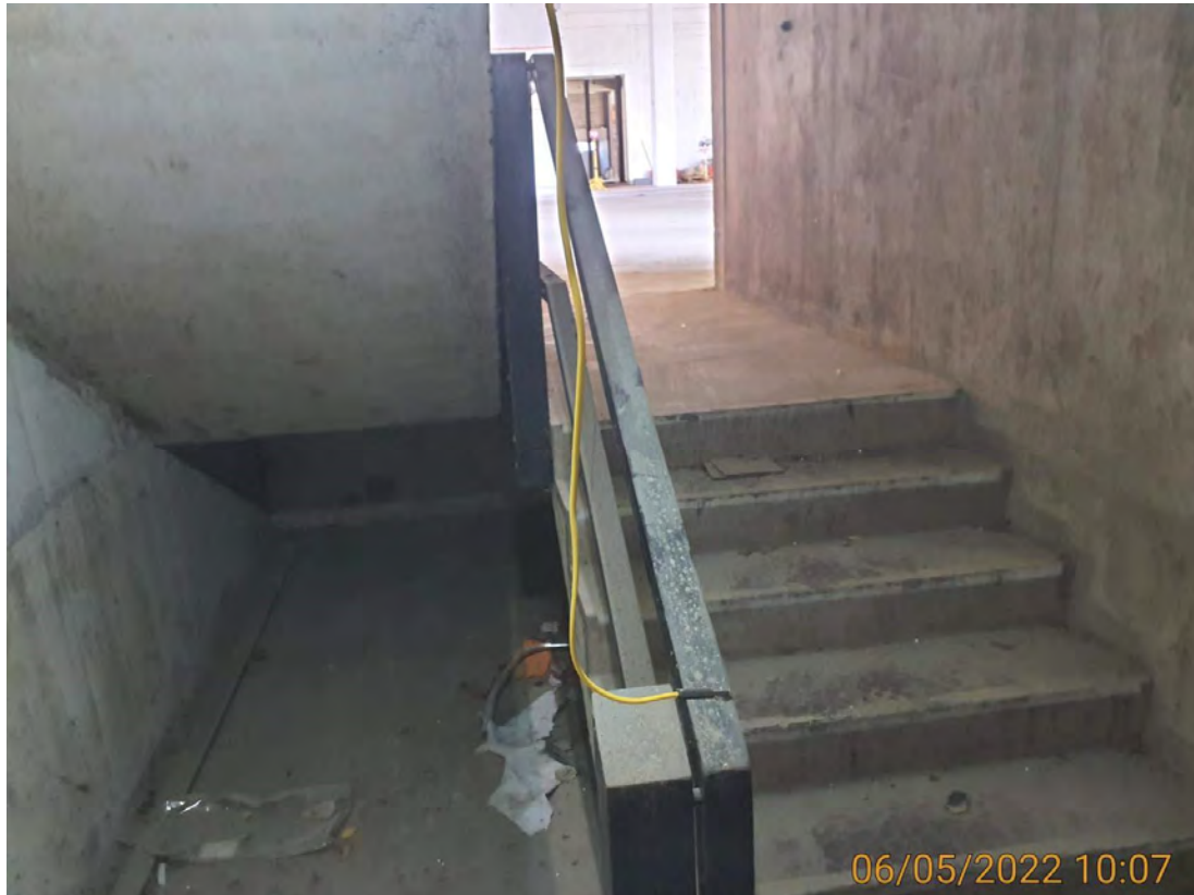
Plate 9 – Lowest level within southern staircase in the southwest corner of the building.
