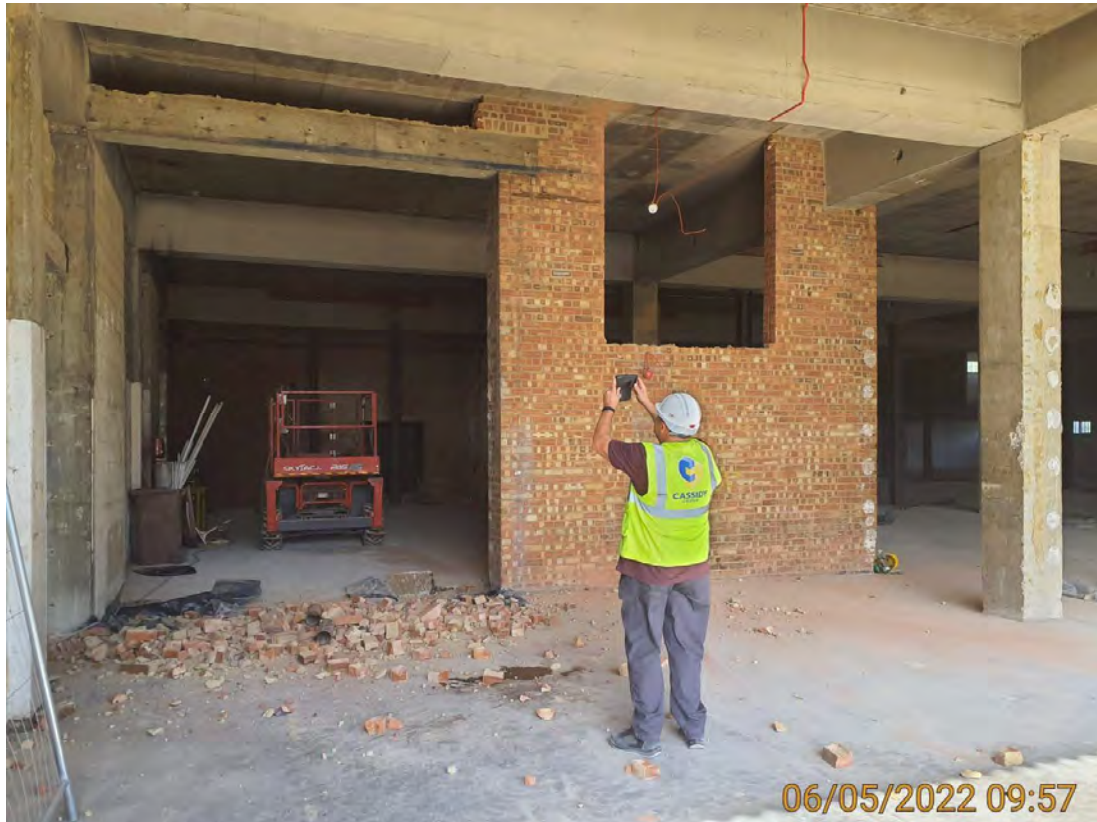
Plate 1 - View into main loading bay.
