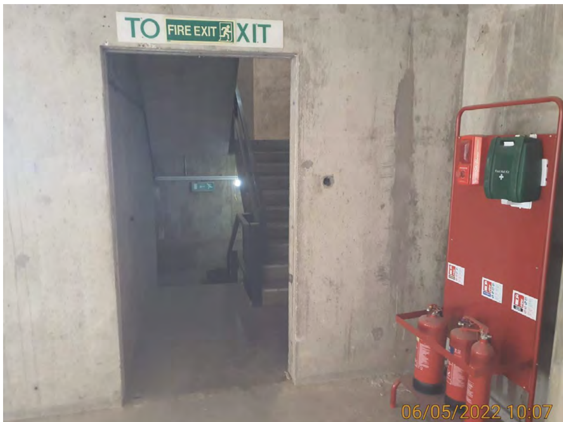
Plate 8 - Southern stairwell in the southwest corner of the building.
