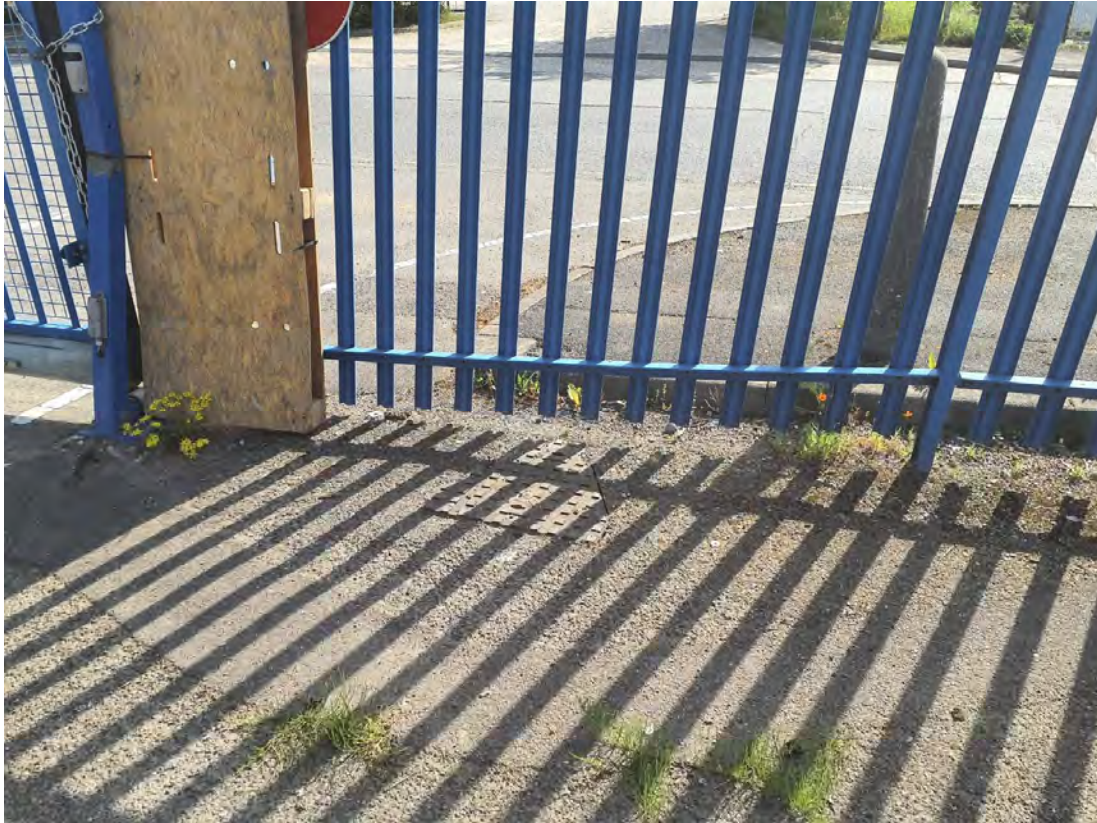
Plate 19 - Manhole cover located in the southeast corner of the site.
