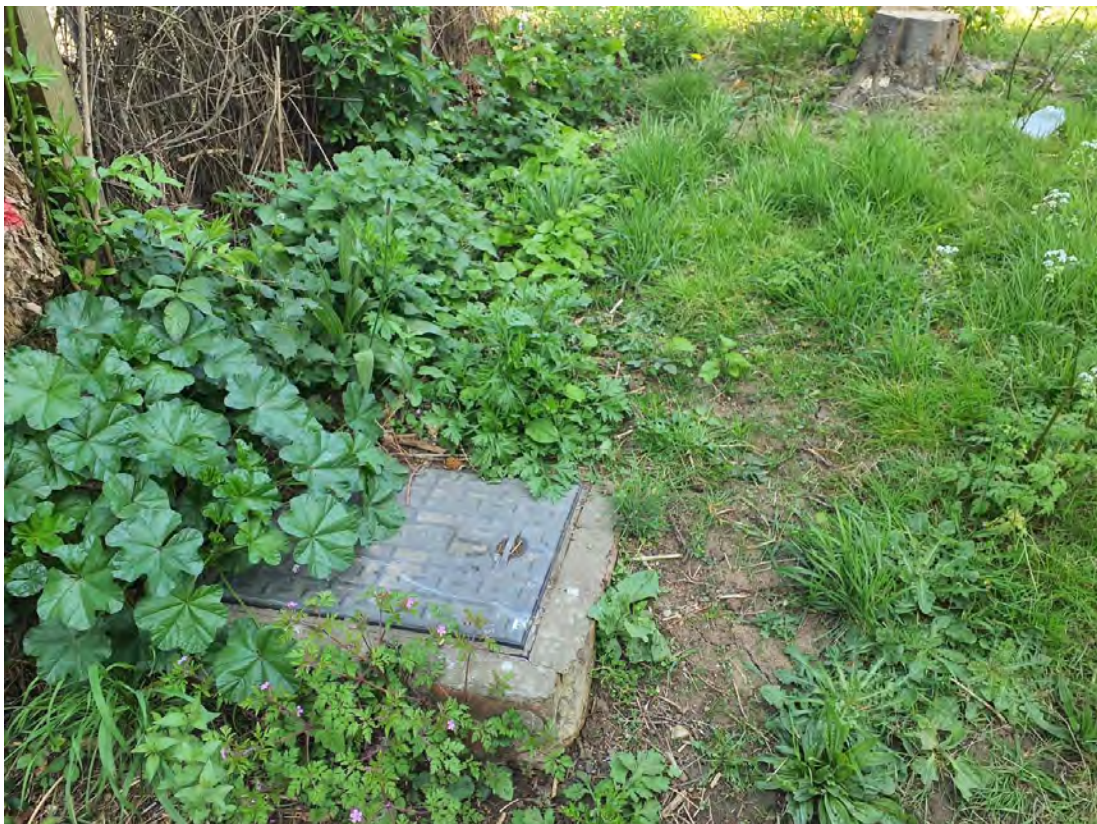
Plate 30 - Manhole cover in the north-western corner of the site.
