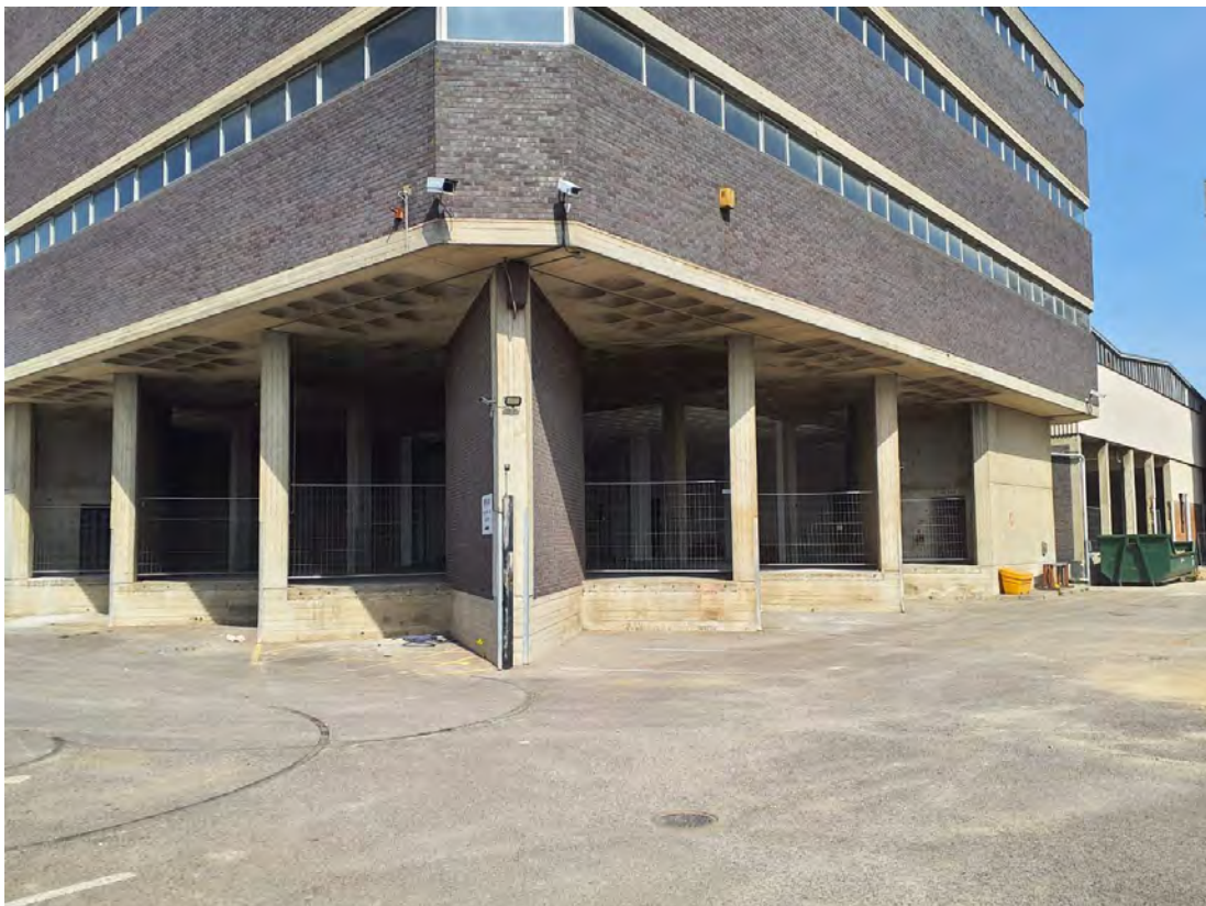
Plate 24 – View of southern loading bays.
