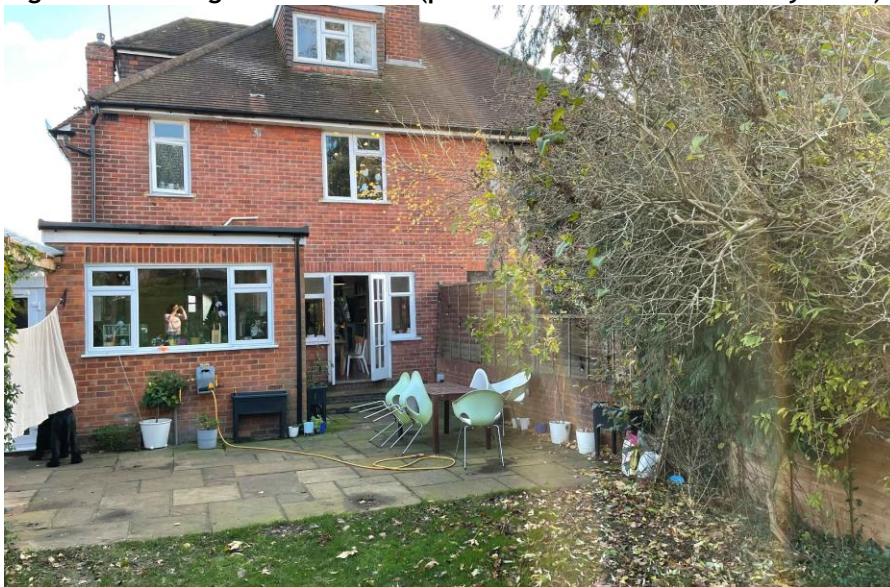
Figure 1: Existing Rear Elevation (photo received on 4 th January 2021)
