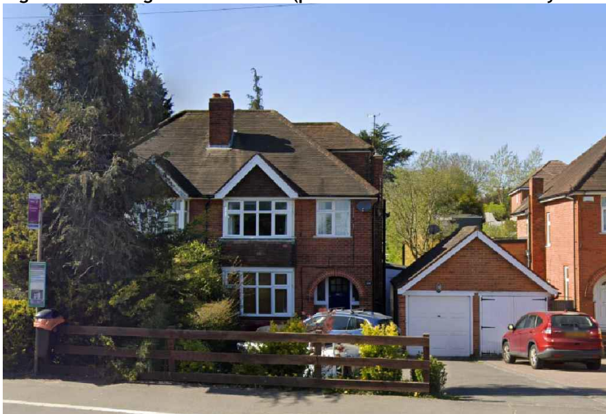
Figure 2: Existing front elevation (photo received on 4 th January 2021)
