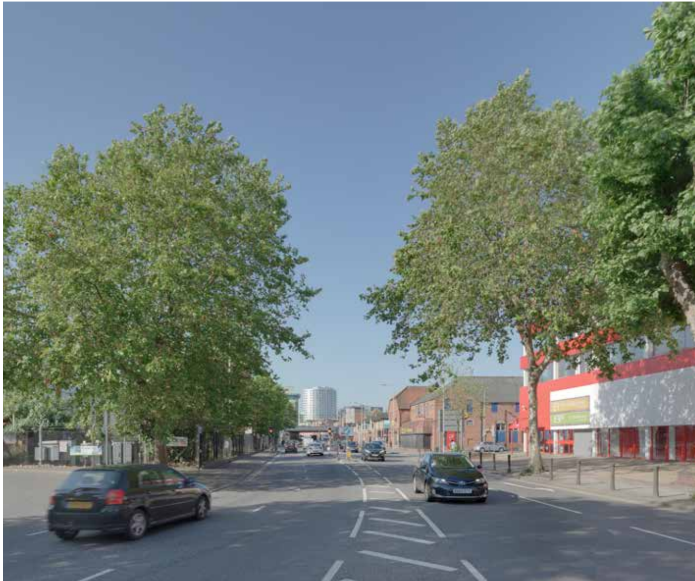
Existing view from Caversham Road Roundabout
