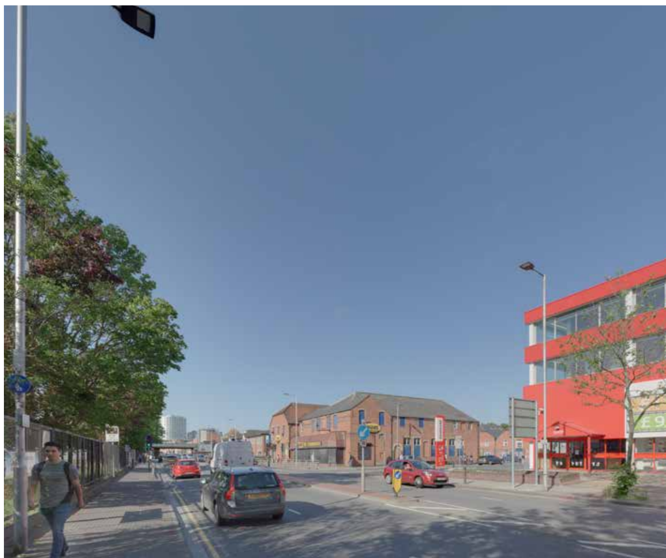
Existing view from Caversham Road north
