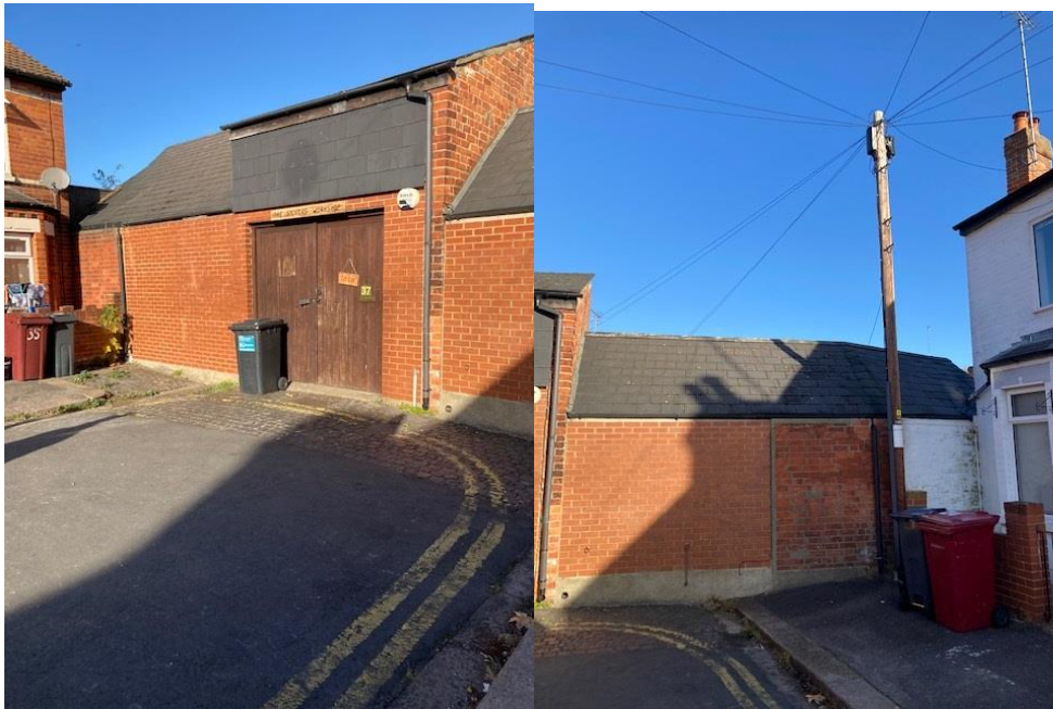
Figure 2 Views of the Site from Hilcot Road
