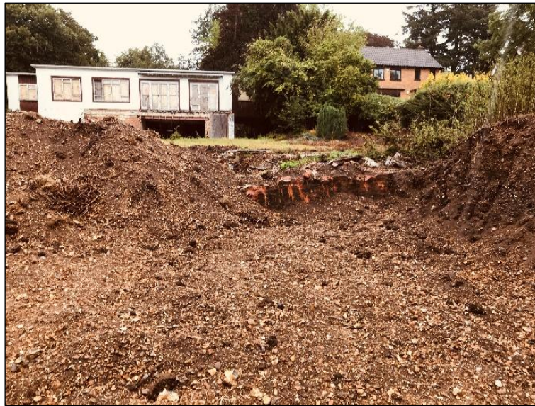
Plate 8. Bare earth in the rear garden (looking north)
