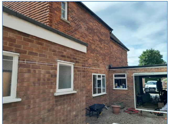
Fig 2. Side of 26 St Peters Hill. Photo taken on 19/08/2022.
