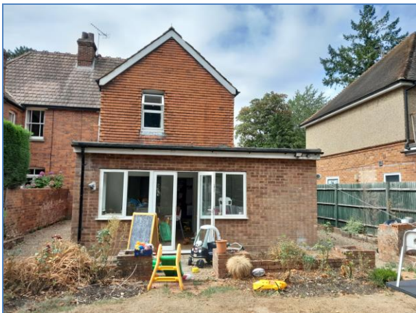
Fig 1. Rear of 26 St Peters Hill. Photo taken on 19/08/2022.
