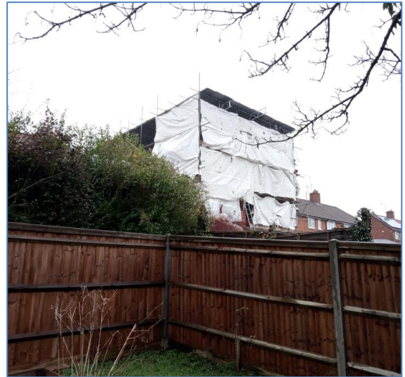
Fig 4. 10 Angelfield Road as viewed from the rear garden of 14 Donkin Hill. Site photo taken by case officer on 02/03/2022
