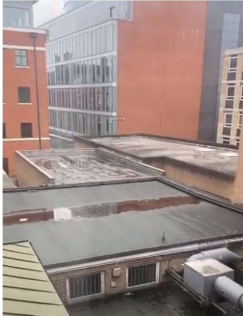
Photograph of the rear of 13 – 16 Market place and the rear additions to be removed.
