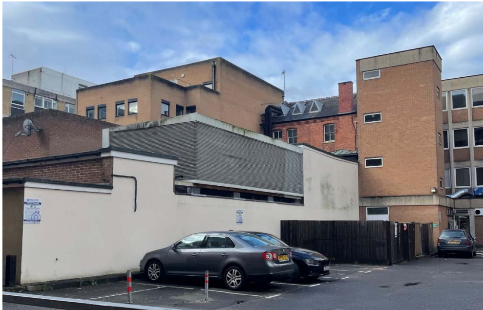
Photograph of the rear of 13 – 16 Market place and the rear additions to be removed.
