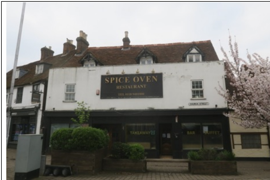
Non symmetrical dormers to principal façade of 2-4 Church Street, Reading.
