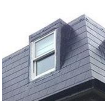
Mansard with Lead Dormer
