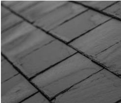
Slate shingle Roof
