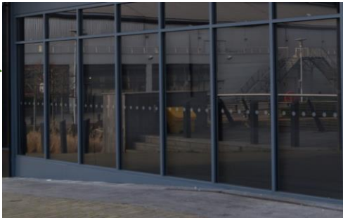
Aluminium Glazed Shop Frontage
