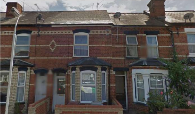
Terrace Housing – Kensington Rd
