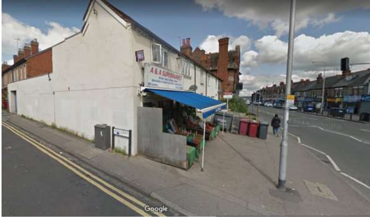
82-84 Whitley Street Google Street View, dated May 2014
