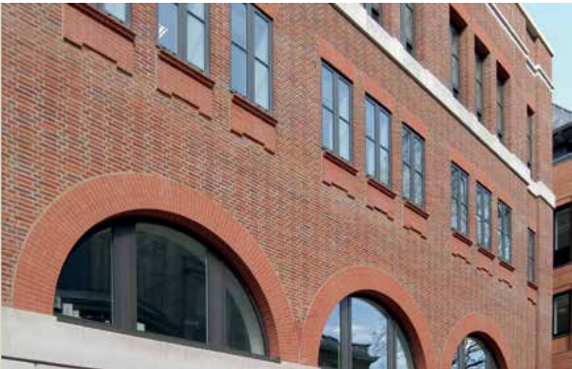
Main brick - Swanage bespoke blend (Handmade Light Red and Restoration Red)
