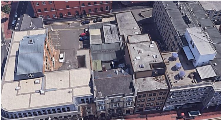
Aerial view looking east
