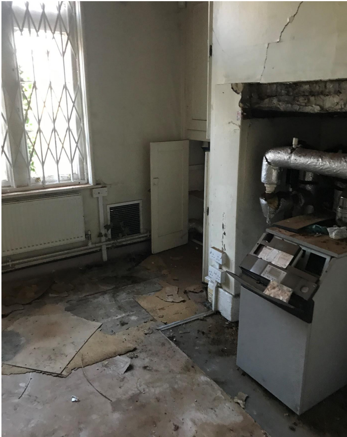
Rear room in front of chimney breast is location for new platform lift
