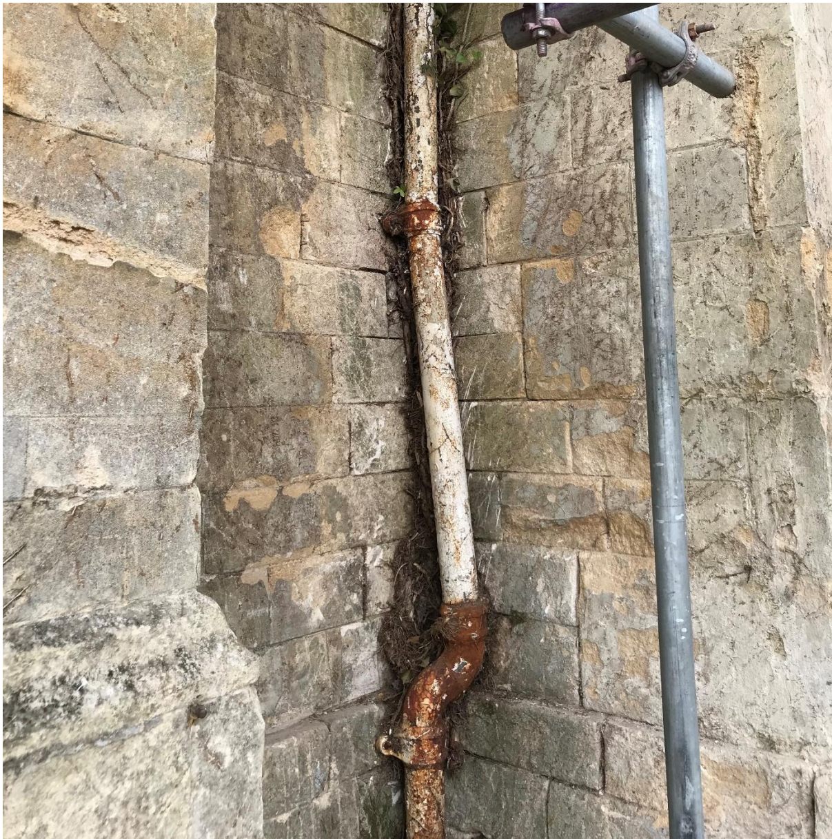
Rainwater pipe to east elevation after ivy has been removed.
