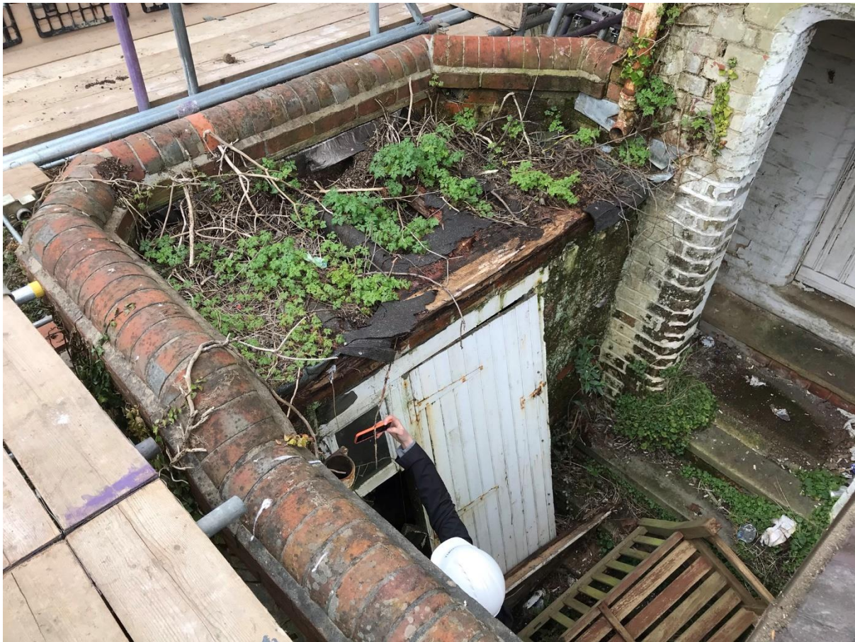
Courtyard area with structure G22 to be demolished. Note rainwater discharge from main roof onto roof of this structure.
