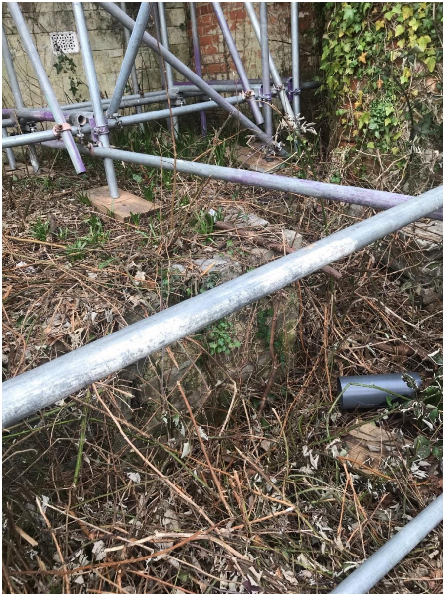
Remains of existing retaining wall
