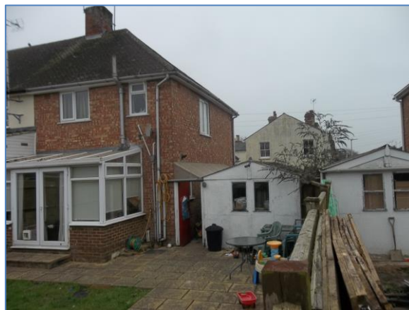
3. Rear of 34 Mill Road. Photo provided by the agent on 26/01/2022.
