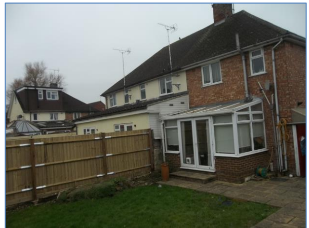
2. Rear of 34 Mill Road. Photo provided by the agent on 26/01/2022.
