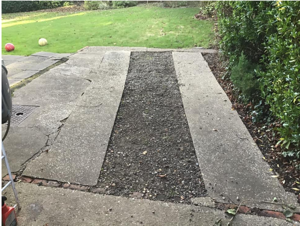
Photo 1: Concrete to be removed from adjacent the new extension location.
