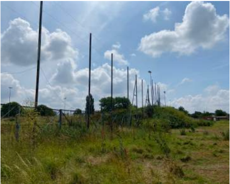
Boundary fence to Rivermead Leisure Complex
