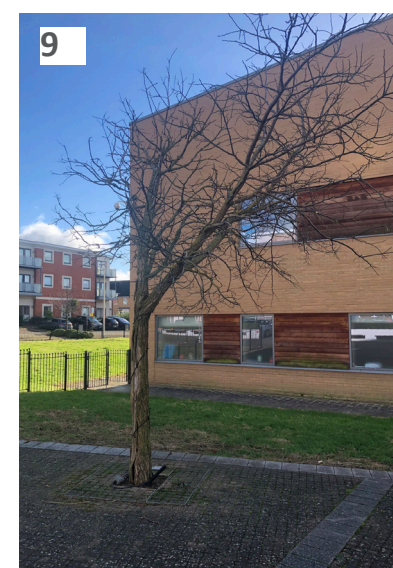
Trees are of poor form and showing dieback, these will be replaced
