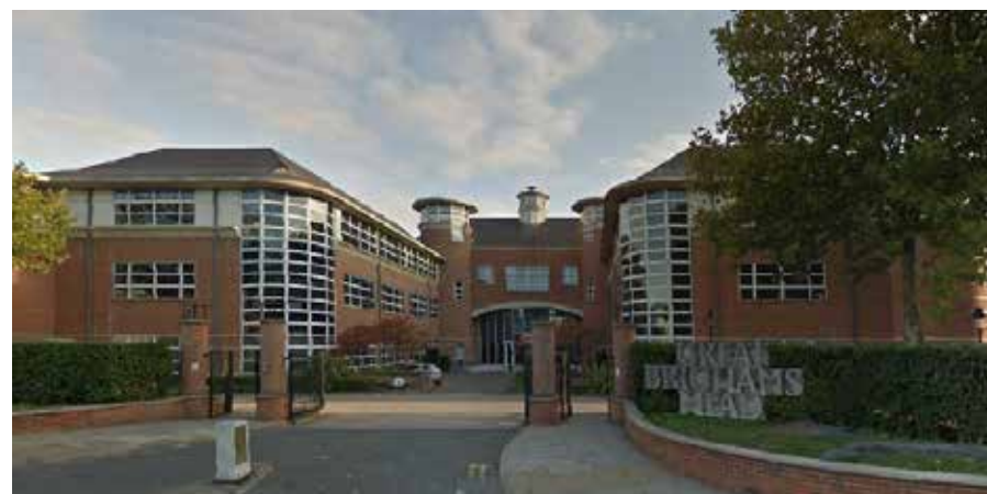
8 View facing onto a 3-Storey office building.
