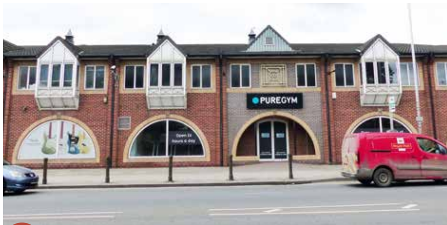
4 View facing onto commercial building on Caversham Road.
