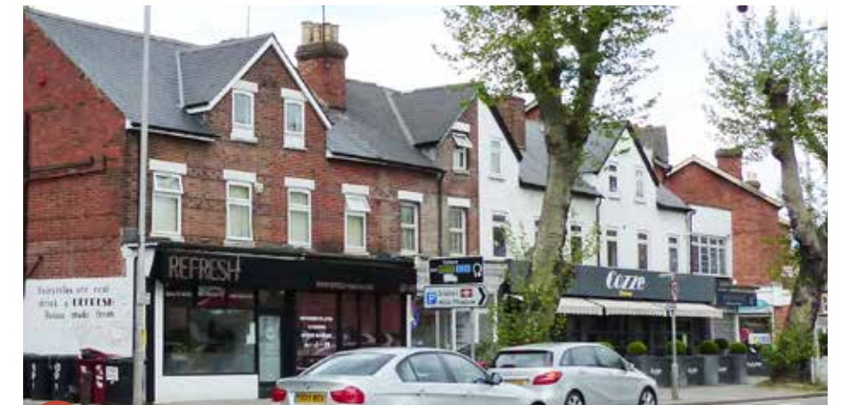
6 View of flats above store fronts.
