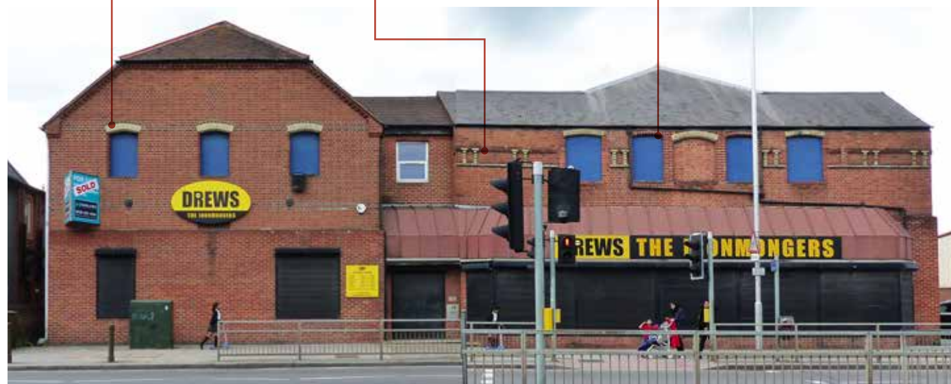
Existing 'Drews' building façade facing Caversham Road
