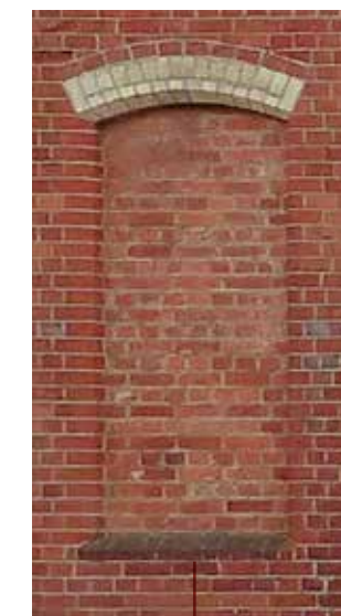
Inset brick to replicate window opening
