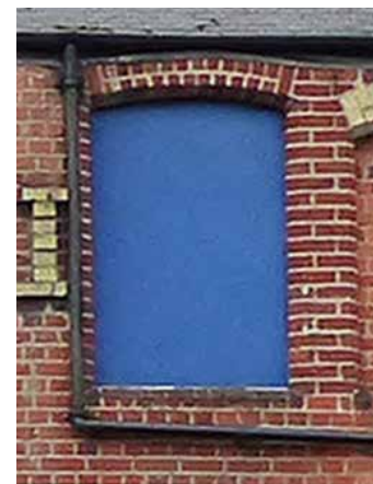
Red brick arch lintel
