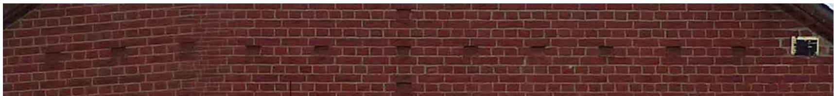
Dentil course brick detailing
