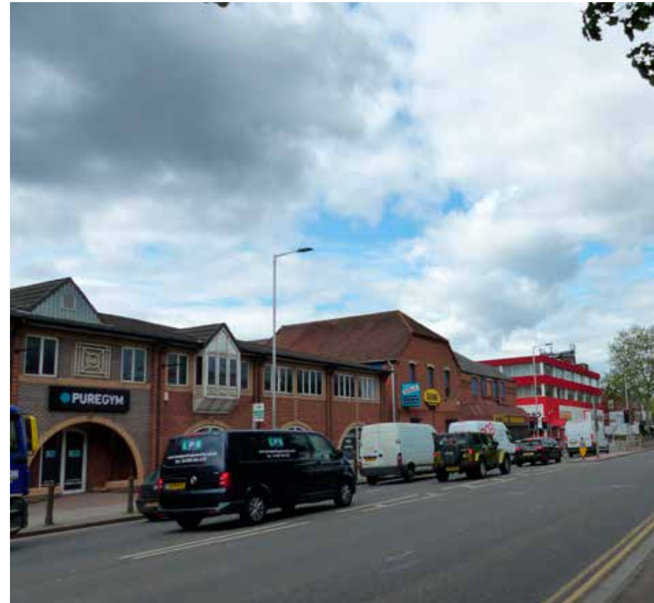
View from Caversham Road showing existing two storey neighbouring commercial building
