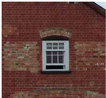
Small sash window with arch lintel
