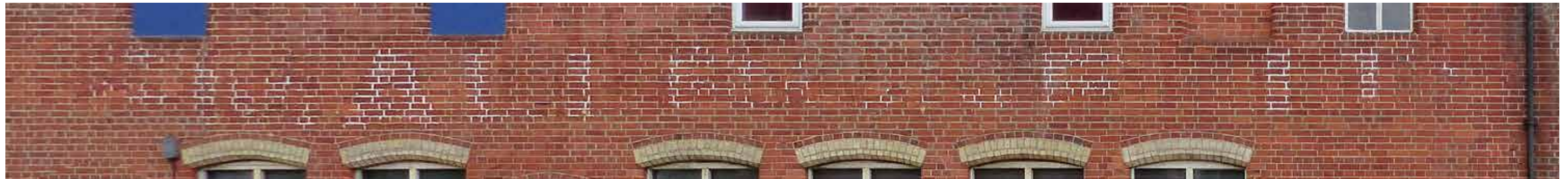
'Ghost' sign-lettering at first floor level on Northfield Road - possibly 'SMALL BONE LTD.'
