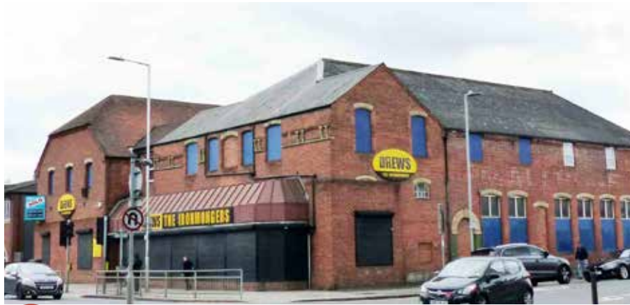
1 View from Caversham Road of the existing building on Site.
