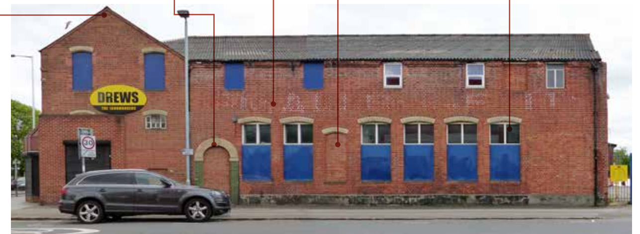
Existing 'Drews' building façade facing Northfield Road
