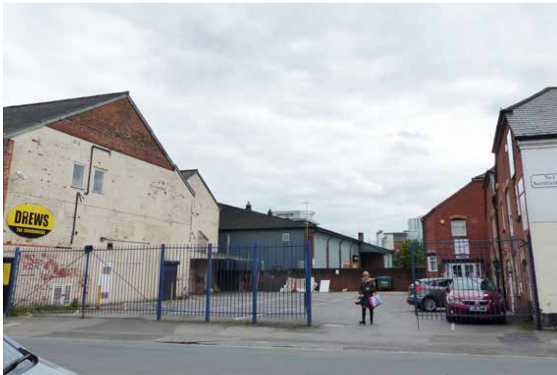
Photo showing poor-quality rear elevations created by the demolition of the rear sections of the building in 1971-1988.
