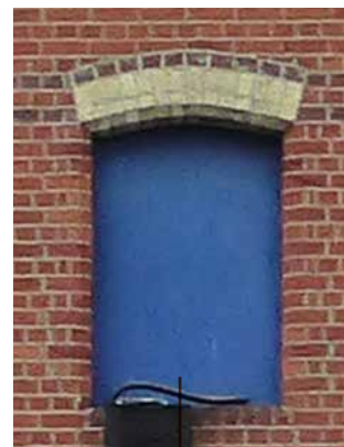
Cream brick arch lintel
