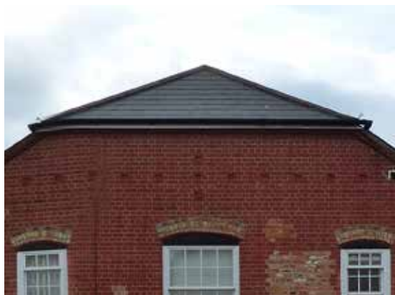
Half hipped roof forms
