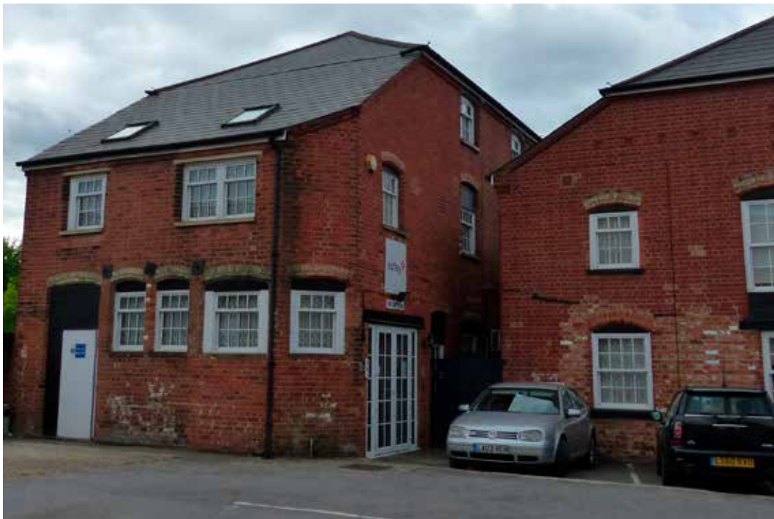
Photo showing existing relationship between the office space and tarmac parking
