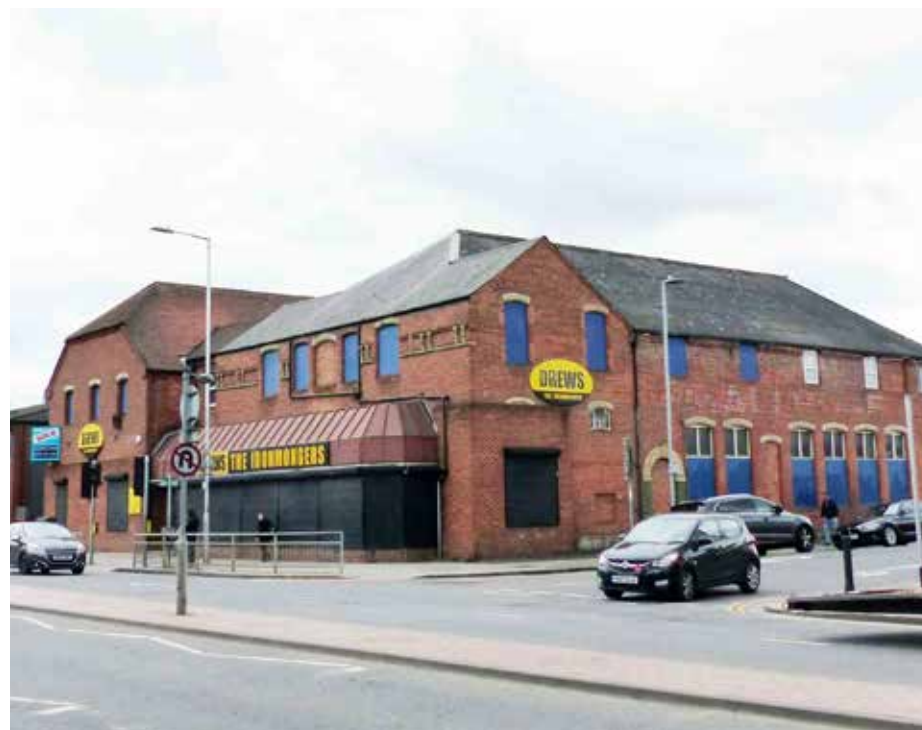
Existing 'Drews' building showing poor relationship between the shop entrance, footpath and Caversham Road
