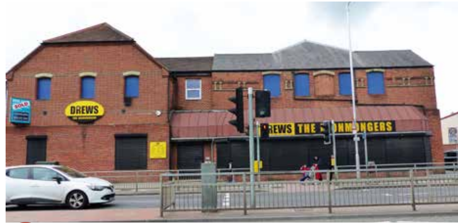
2 View from Caversham Road of the existing building on Site.
