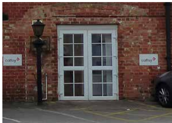
Former arch and now turned into a double door with brickwork infill
