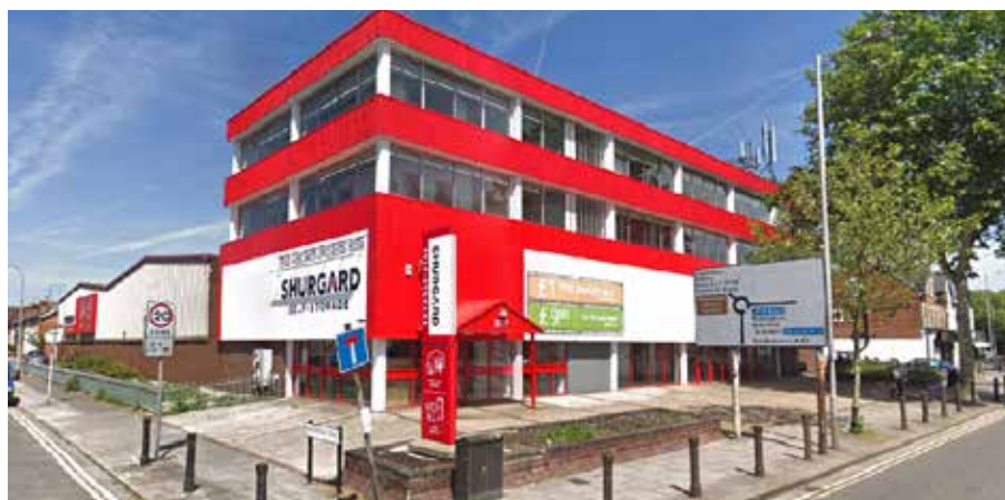
7 View facing onto a 3-Storey office building.
