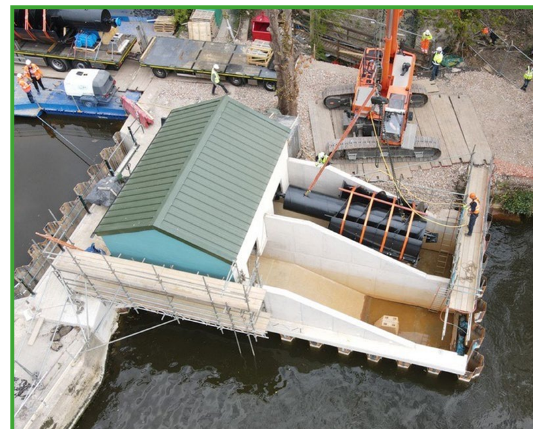
The turbines being installed
