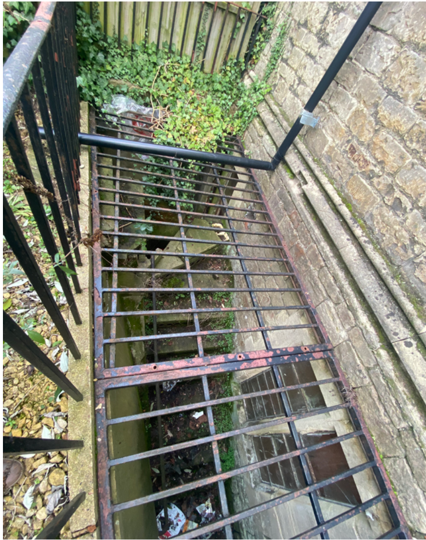
Fig. 17: Photograph of stepped access lightwell owned by Reading Borough Council
