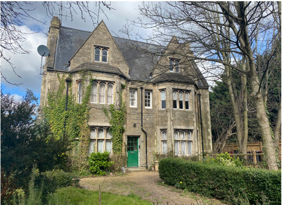
Fig.12: View of south elevation with non-original central entrance door and windows
