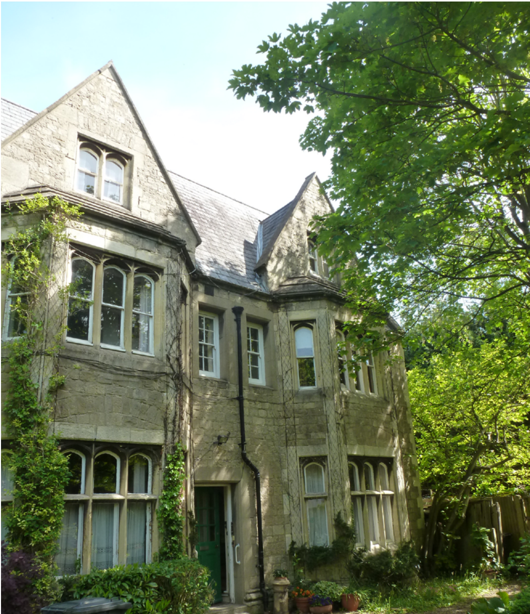
Fig.2: Existing view of Carlisle House from the south
