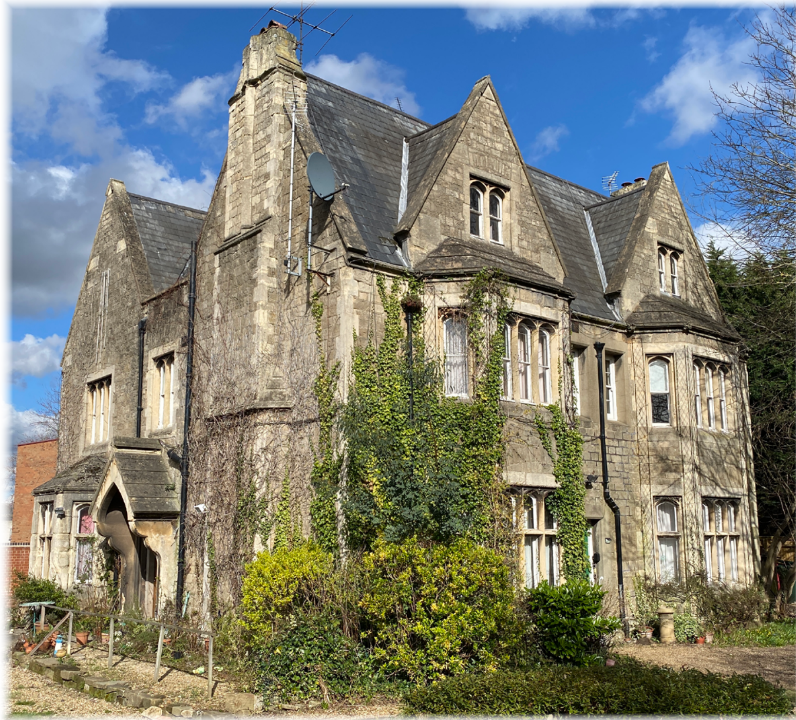
Fig.1: Existing view of Carlisle House from the south-west
