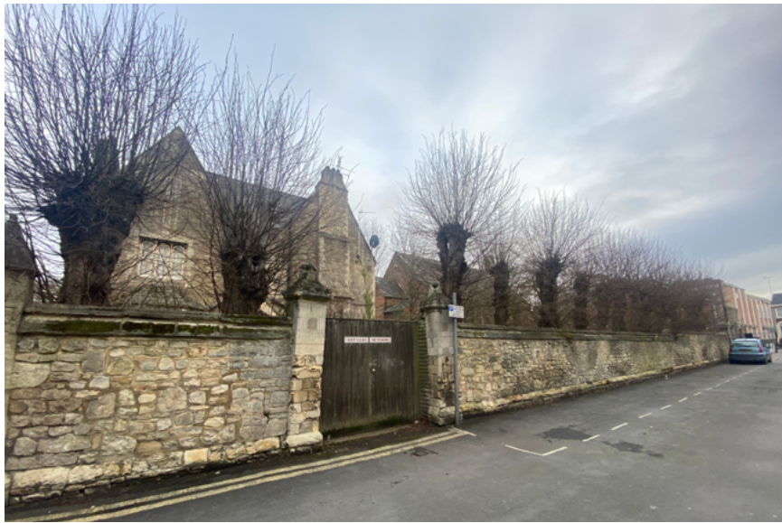
Fig.7: View of western boundary with Trinity Place and vehicle access gates which are to be replaced.
