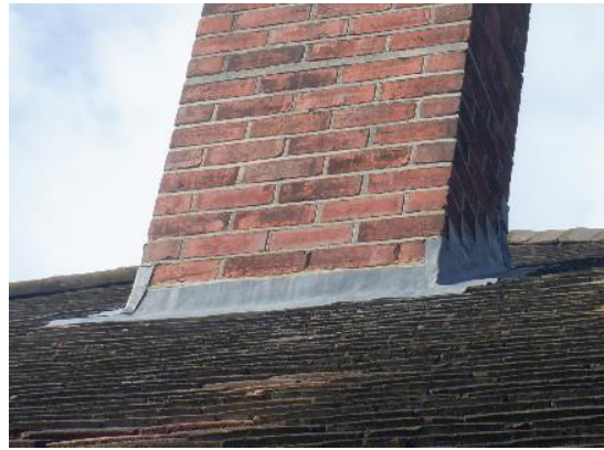
8. Tight lead flashing around chimney.
