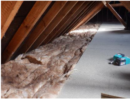
13. Boarded floor with fibreglass insulation along the edge.
