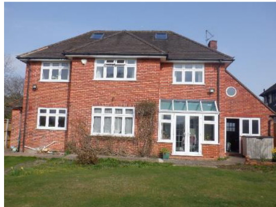
2. Rear of the house viewed from the west.
