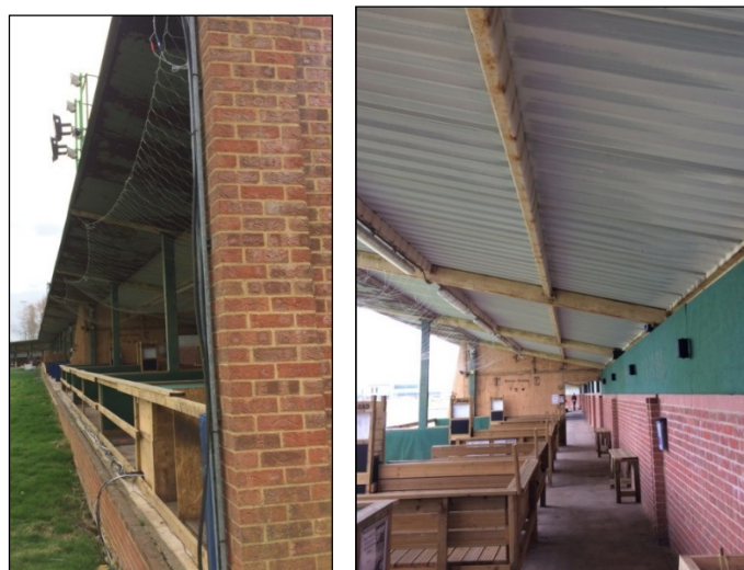
Figure 6 Building to the north of the stream at Richfield Avenue
