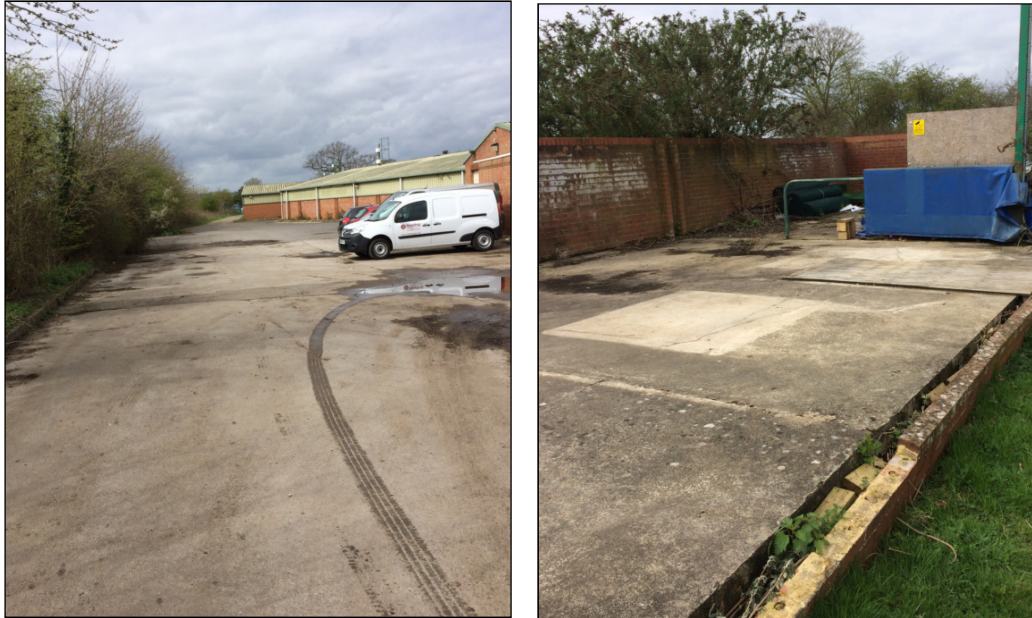
Figure 5 Car parking to the south of the building (left) and area of hardstanding on site of demolished building (right)
