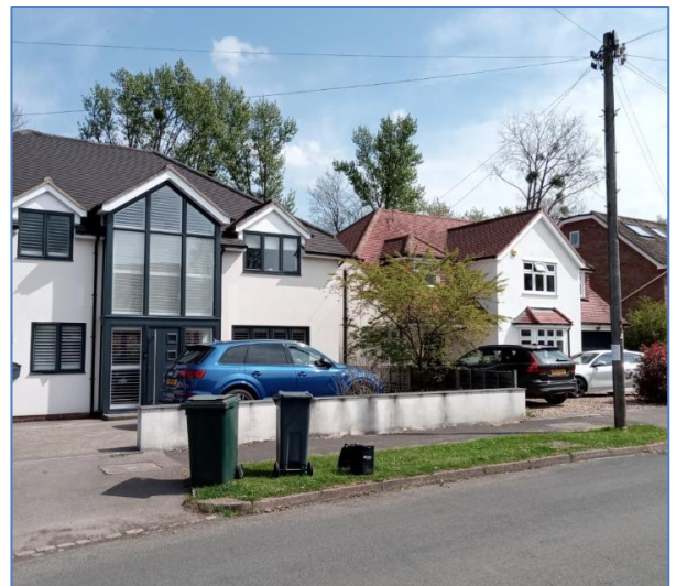
2. Rear of 9 Eric Avenue. Photo taken by case officer on 20/04/2022.
