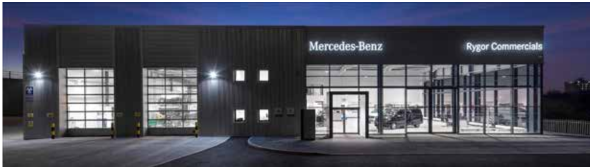
Rygor Commercial Vehicles Sales and Workshop facility
