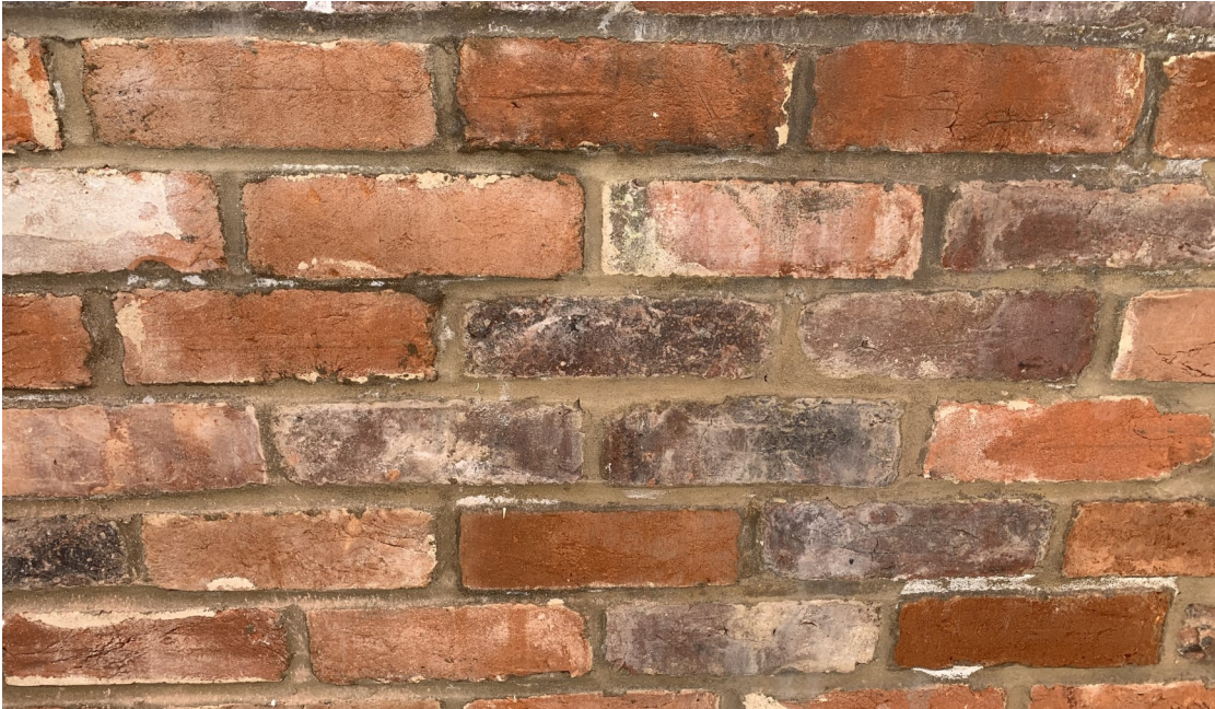
Fig 1767.02 close up of the bricks
