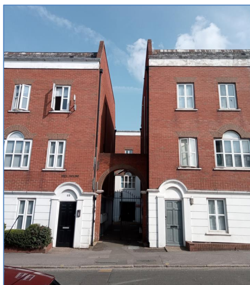
Fig 1 - Front of 87 Southampton Street (in the background) taken by case officer on 25/03/2022
