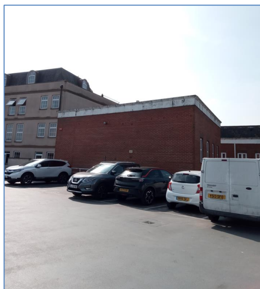
Fig 2 - Rear of 87 Southampton Street taken by case officer on 25/03/2022
