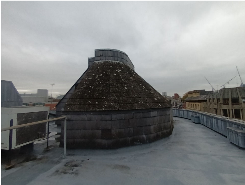
Photo 1. The plant room structure
