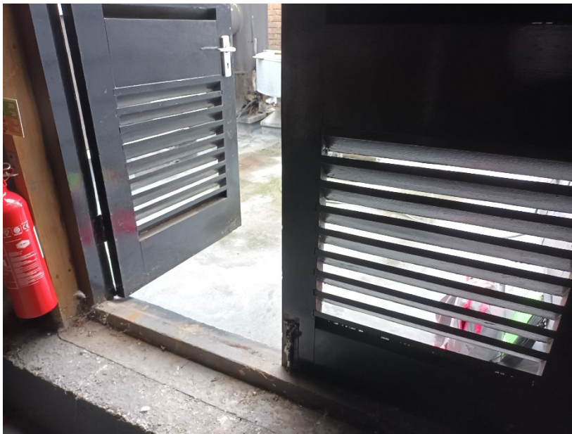
Photo 7. Slatted doors allowing possible bat access to the interior
