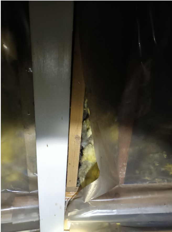
Photo 10. Example of potential roost space between timber batons and insulation layer
