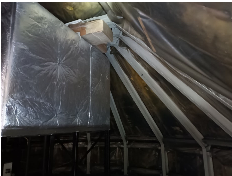
Photo 8. Interior. Steel beams with a fiberglass insulation layer with timber batons and a plastic sheeting layer
