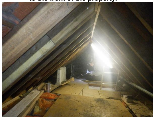
12. Internal view of the roof space boarded at the front southwestern end.
