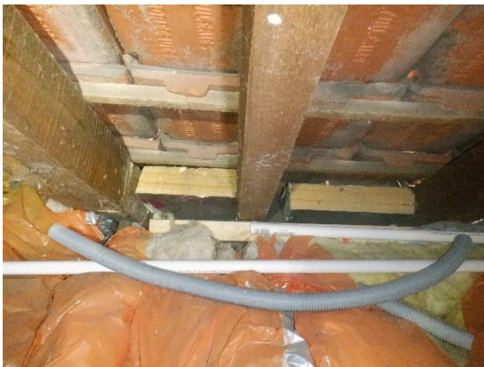
15. Eaves filled with foil-covered insulation boards in places.
