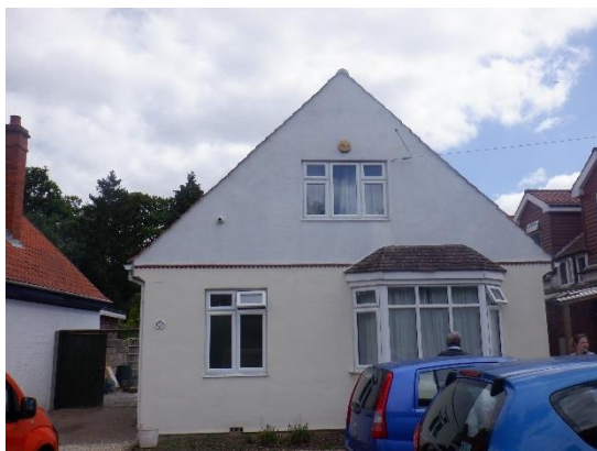
1. Front of the bungalow viewed from the southwest.
