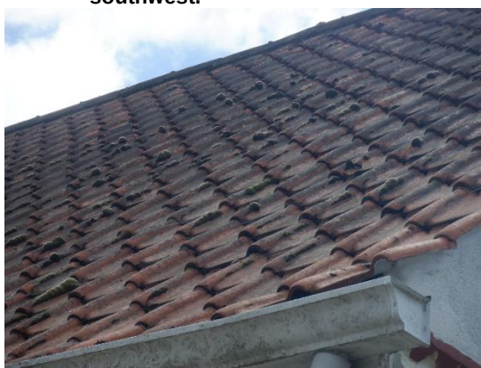
3. Interlocking roof tiles in place and tightly fitted.
