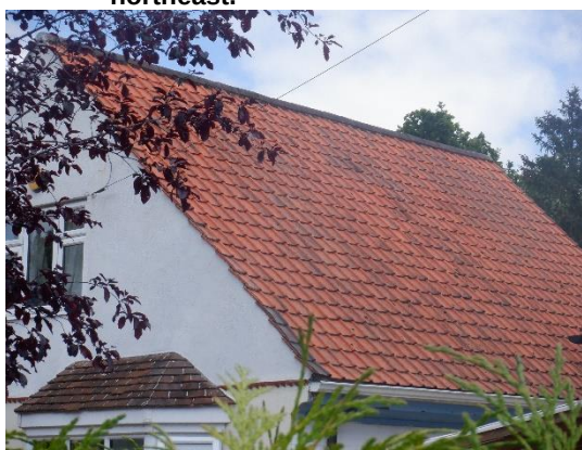
4. Ridge tiles in place and mortared.
