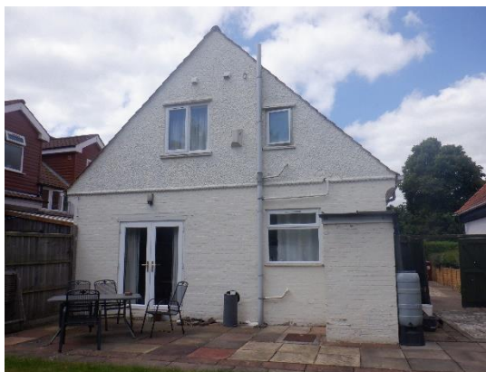
2. Rear of the bungalow viewed from the northeast.
