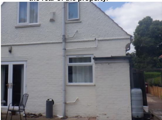
11. Single-storey rear extension tightly fitted.
