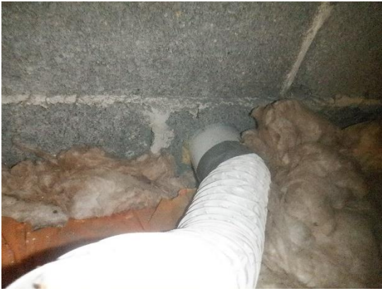
19. Sealed ventilation ducts in the wall of the northeastern gable end wall.
