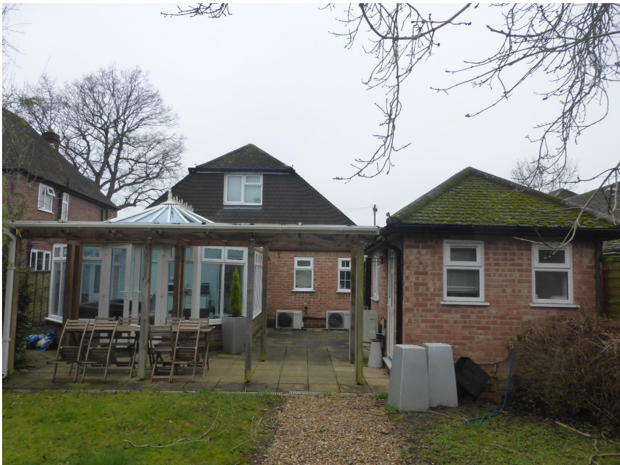
Conservatory, Covered Walkway & Office Outbuilding to be demolished
