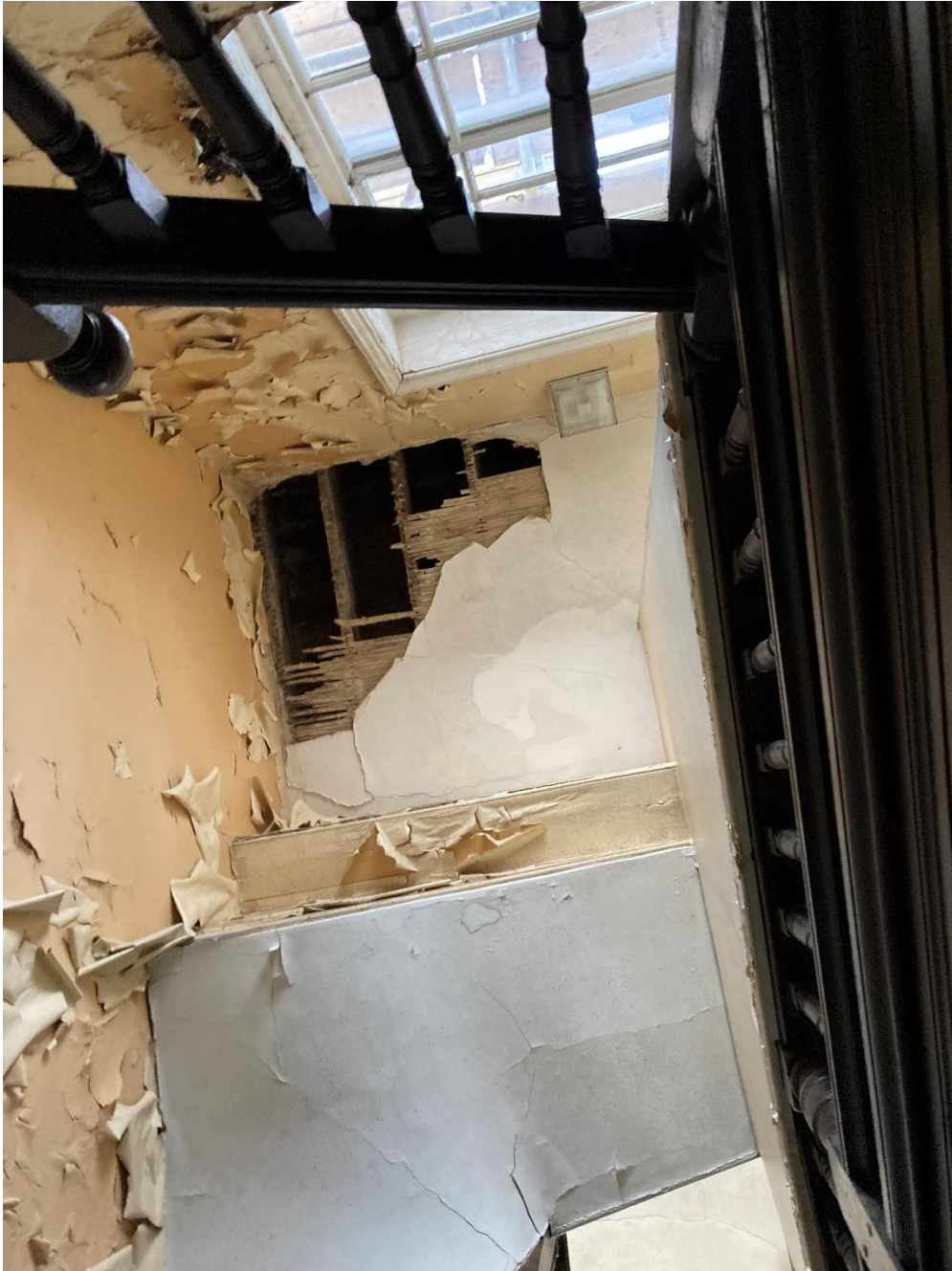
Ceiling over main stair
