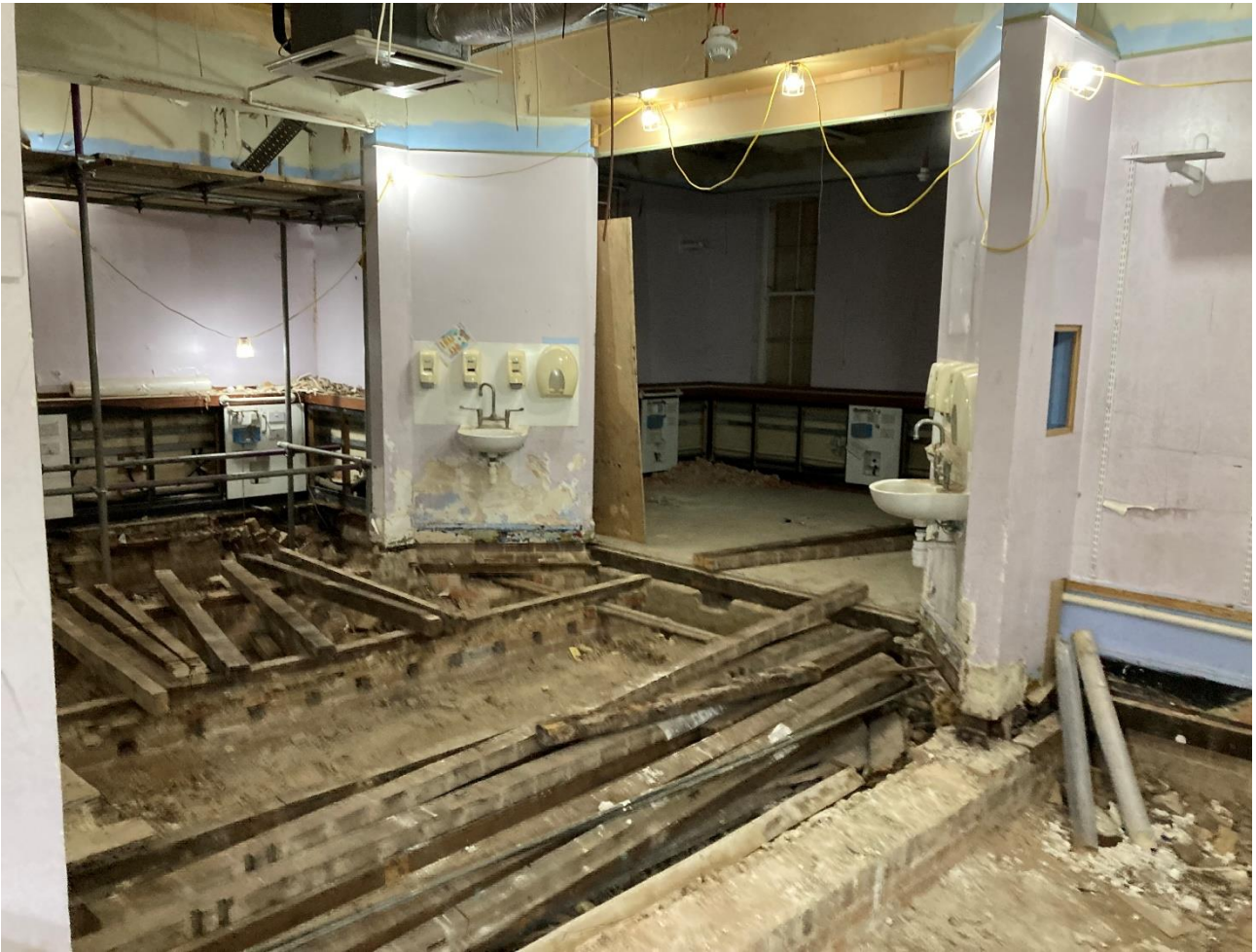
Timber suspended ground floor and concrete beyond
