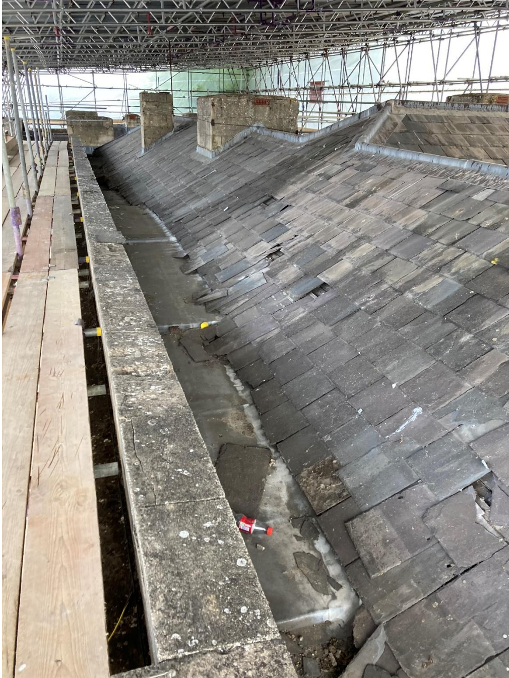
General view of the roof
