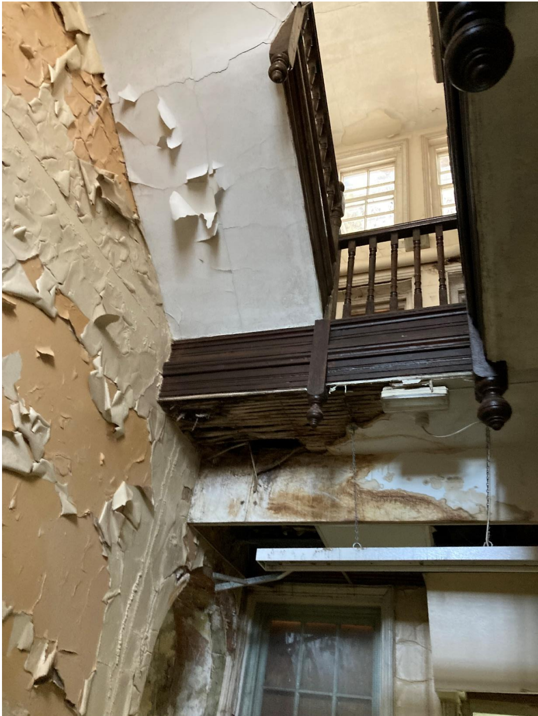
First floor landing (inaccessible)
