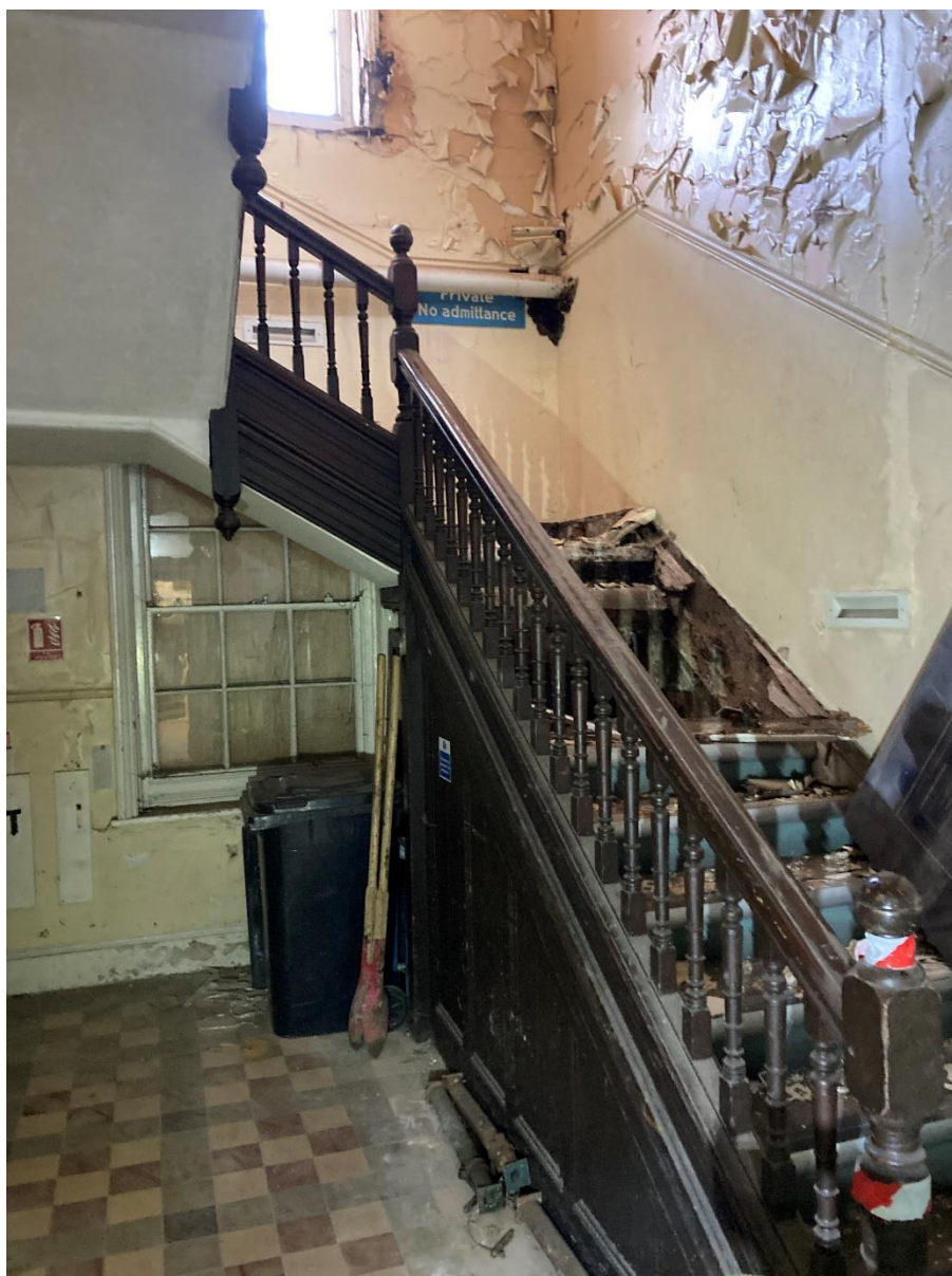
General view of the staircase at ground floor
