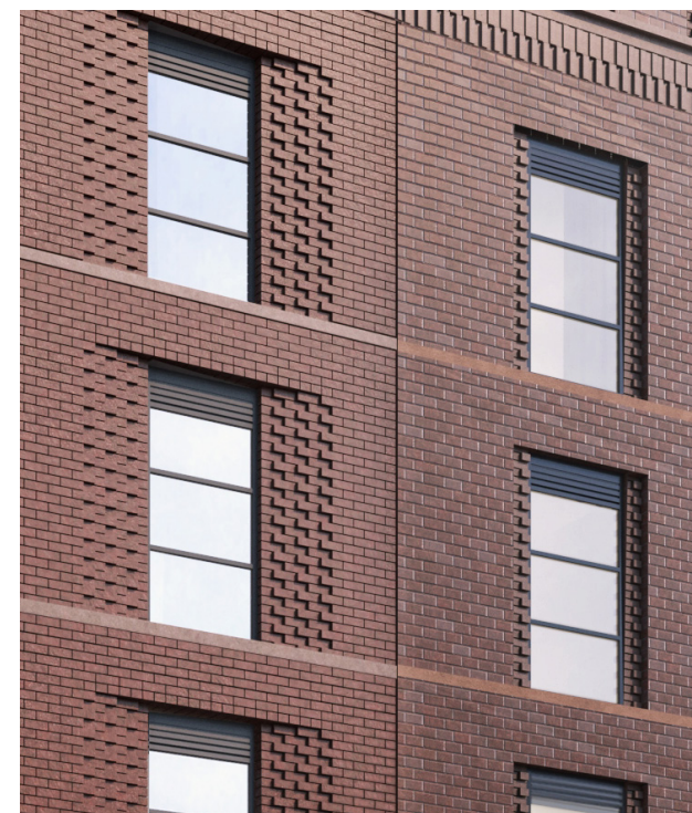
Figure 6.11 Details of brick work [taken from DAS by FCH Architects]
