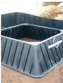
Root Director RD1400A during installation
