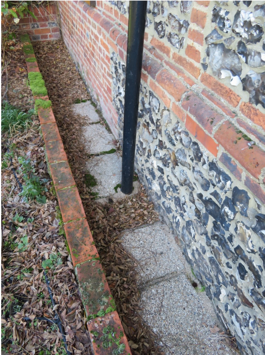
Image 8: Hard Cementitious Mortar at Low-Level to Front Elevation
