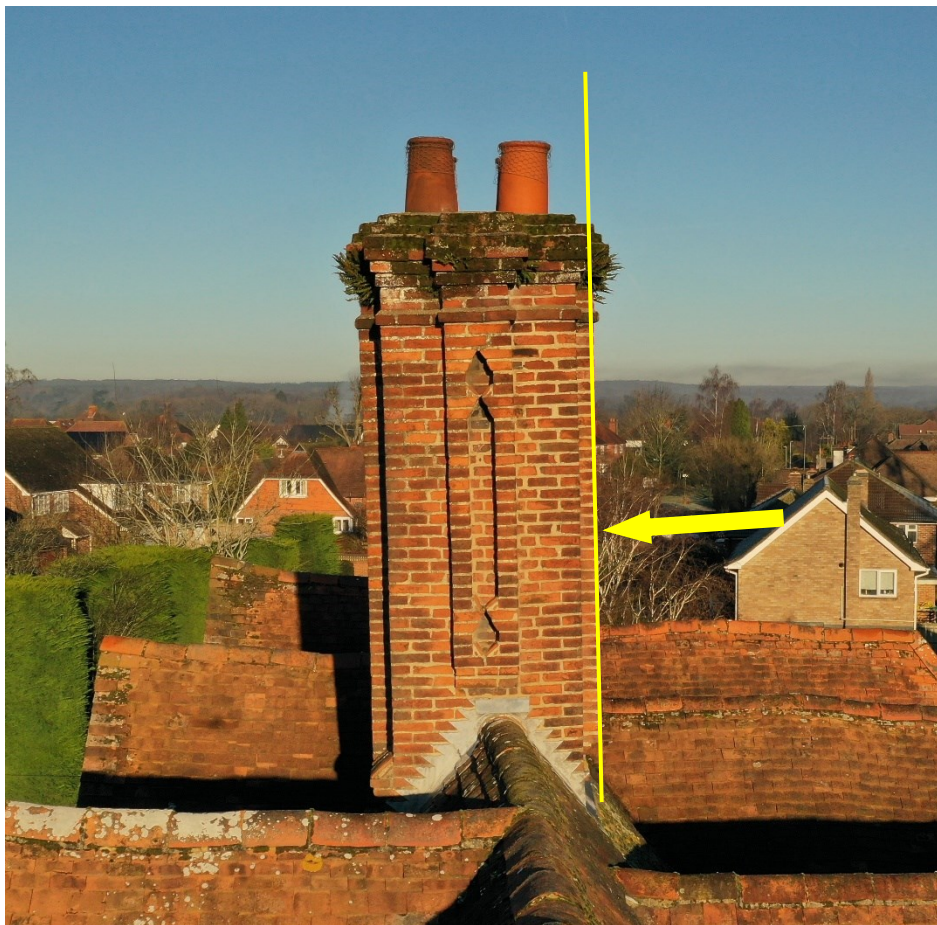
Image 4: Lean to Central Stack
