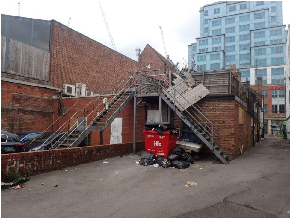
Photograph 10: Fife Court on the site at Friar Street, Reading.
