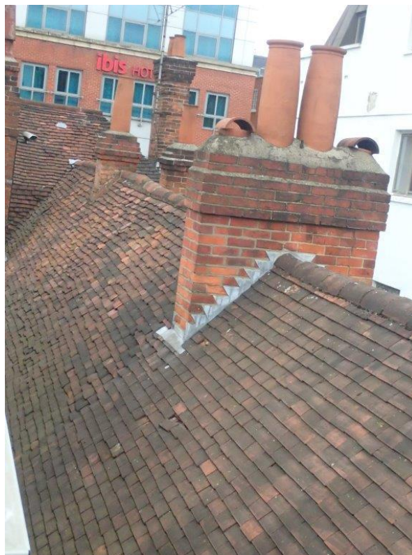
Photograph 8: Roof on the site at Friar Street, Reading.
