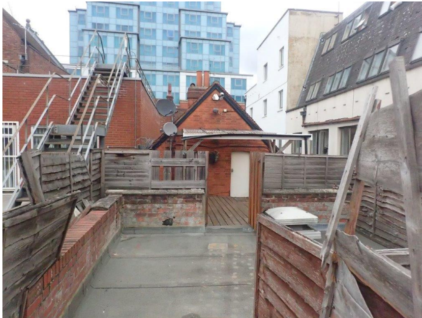
Photograph 7: Roof area on the site at Friar Street, Reading.
