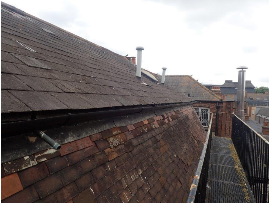
Photograph 3: Roof of buildings on the site at Friar Street, Reading.
