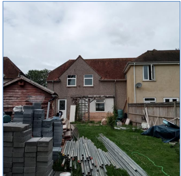
2. Rear of 33 Linden Road. Photo taken on 09/06/2022.
